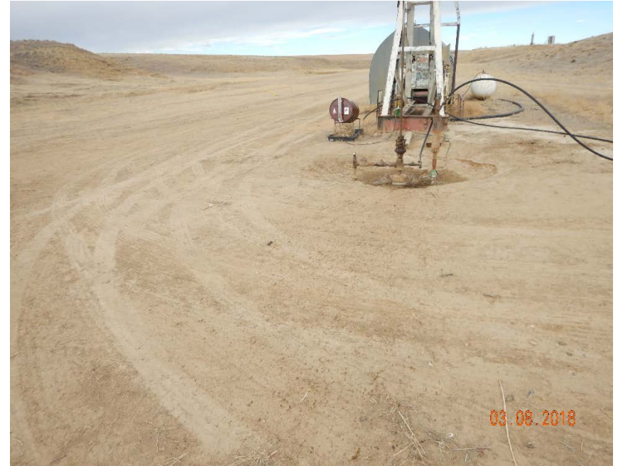
Photo #4 – View from south of SE extent of oily waste spray from wellhead.
