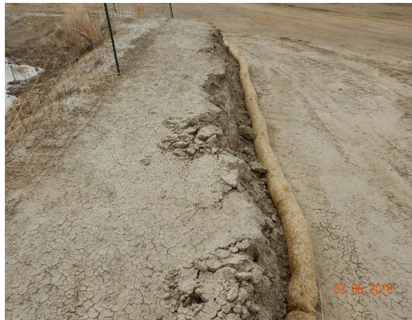
Photo #16 – Straw waddle has been installed along west berm of produced water pit.
