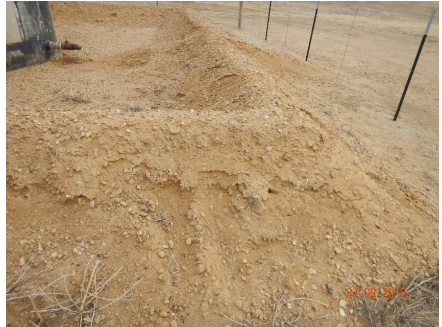
Photo #8 – Eroded pit berm. Note accumulation of oily waste beneath valve (on SE side of crude oil AST).
