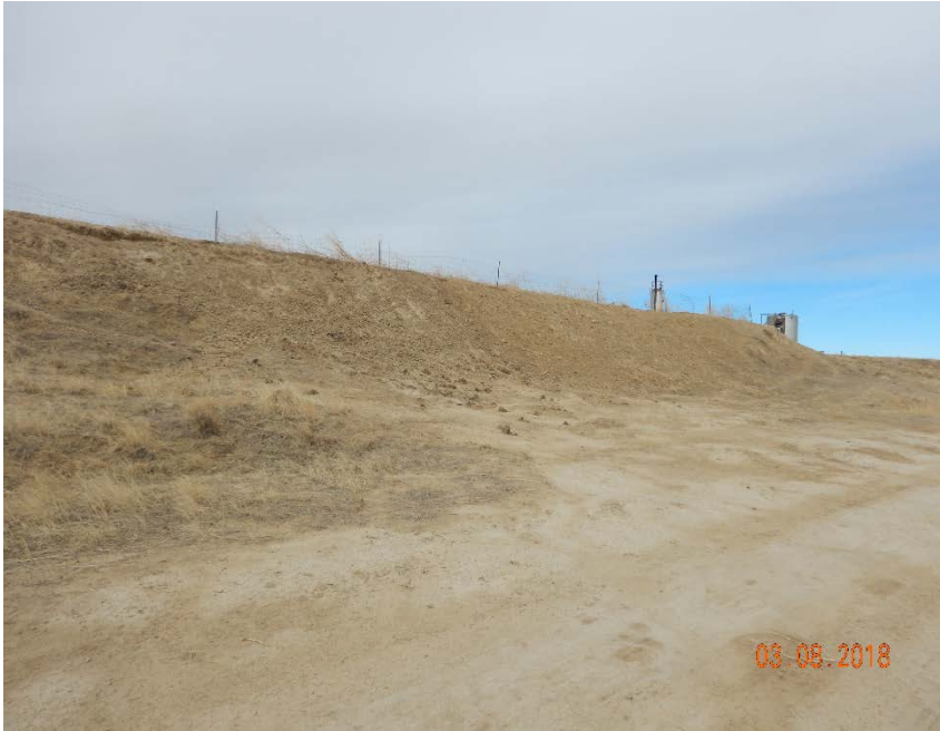
Photo #21 – View of east produced water pit berm. Note evidence of sediment transport and absence of straw wattle.
