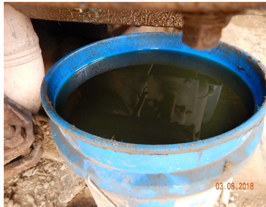
Photo #6 – 5-gallon bucket beneath prime mover is being used to catch used motor oil.
