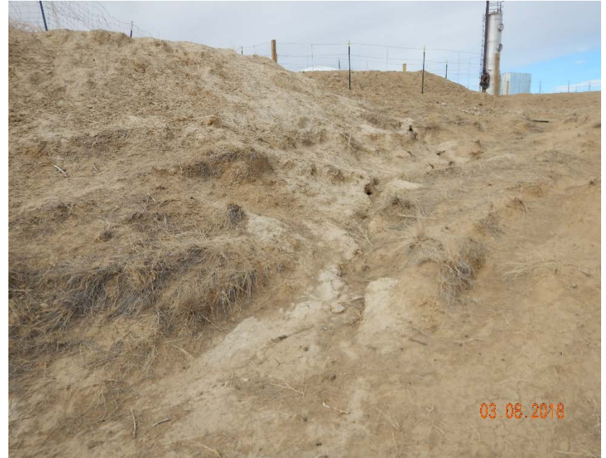
Photo #22 – Erosion and sediment transport at NE corner of produced water pit.
