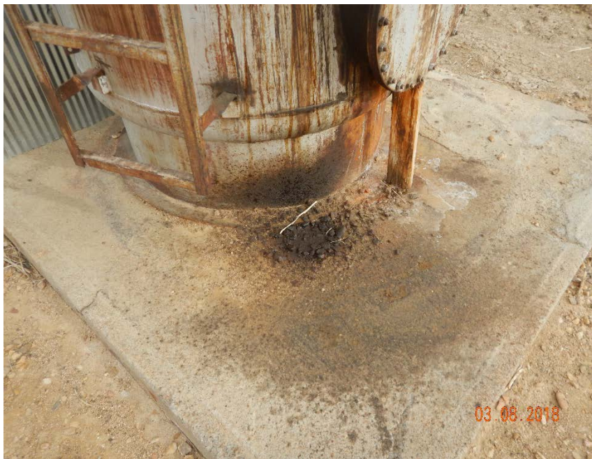
Photo #11 – Accumulation of oily waste on SE side of VHT.
