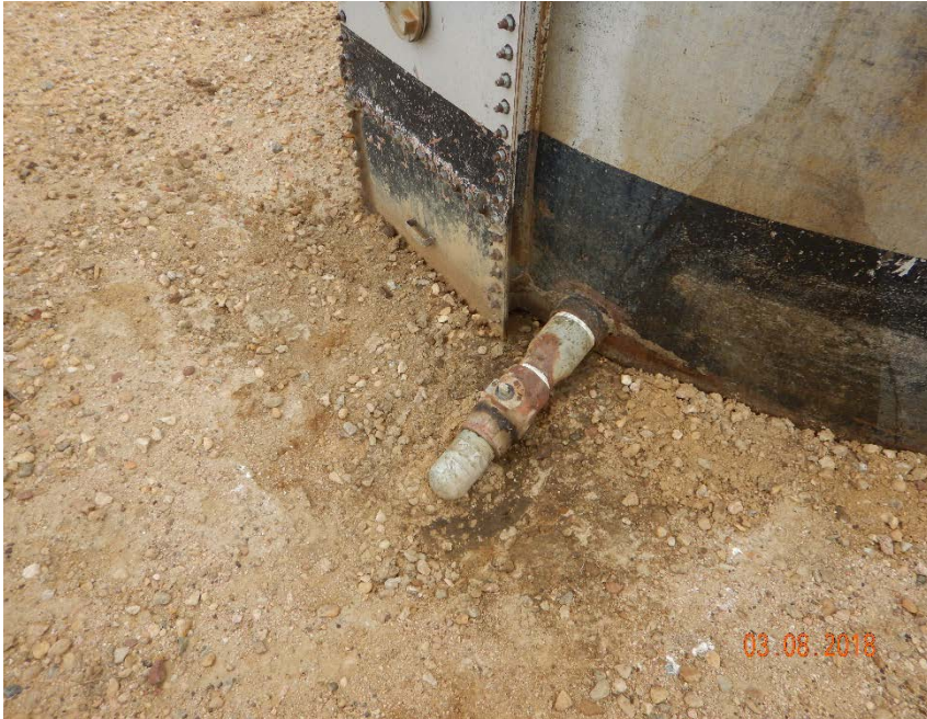
Photo #9 – Accumulation of oily waste beneath valve on NW side of crude oil AST.
