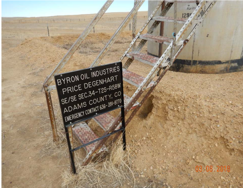
Photo #7 – Battery sign. Note eroded/damaged pit berm and uncontrolled weed growth.
