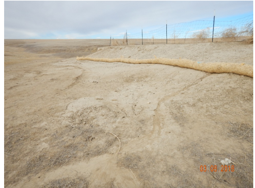
Photo #20 - Straw wattle extending along south berm of produced water pit.
