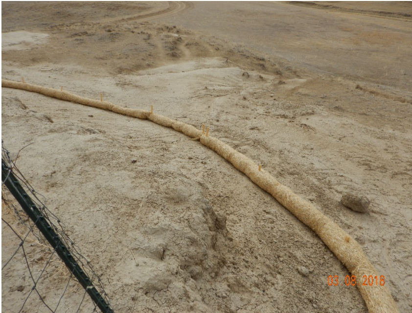
Photo #19 – View of straw wattle at SW corner of produced water pit.
