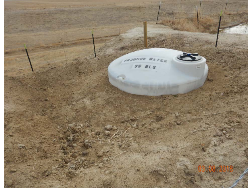
Photo #14 – Skim tank lacks NFPA placard. Earthen berm is insufficient to contain pit contents plus precipitation.
