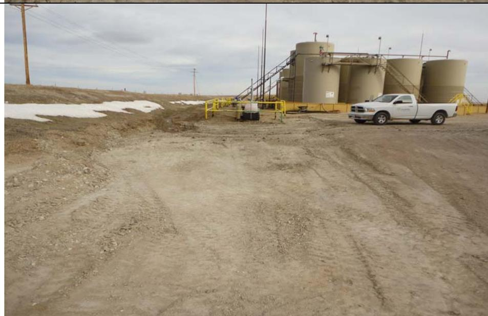
**Subject:** M&E had removed the impacted soils west of the aboveground piping run along the northwest side of the site using a skid steer.
