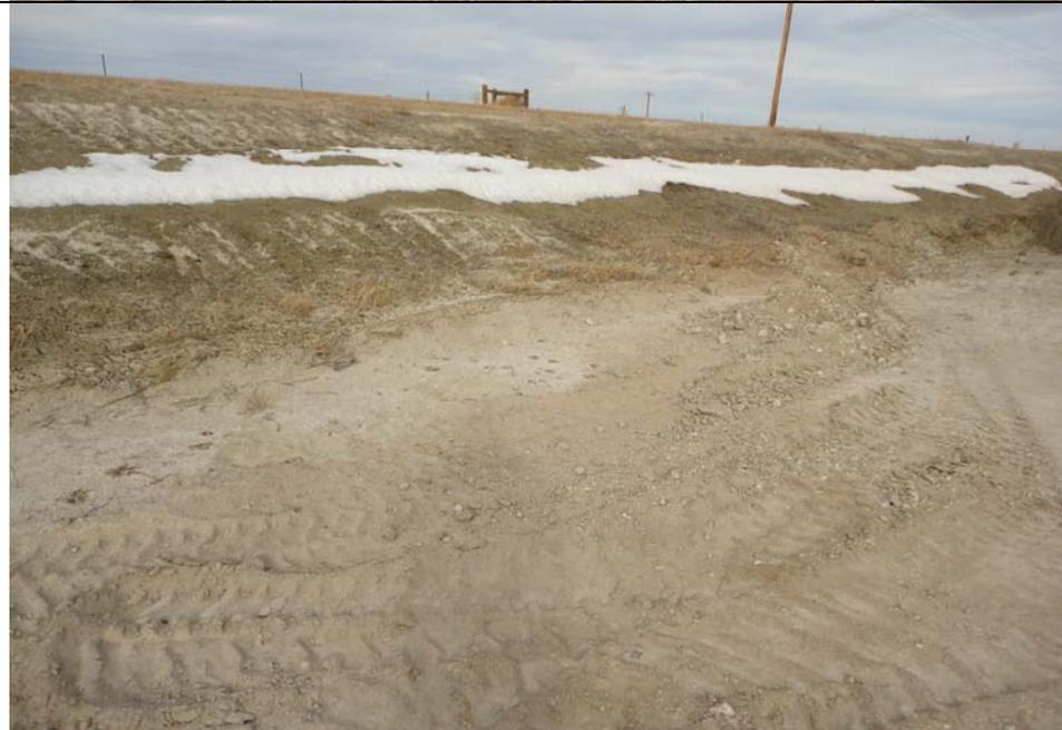
**Subject:** M&E removed the impacted soil along the north side of the Horsetail 19N pad to the west of the piping and base of the north berm. Shallow claystone or siltstone bedrock was present near the surface.
