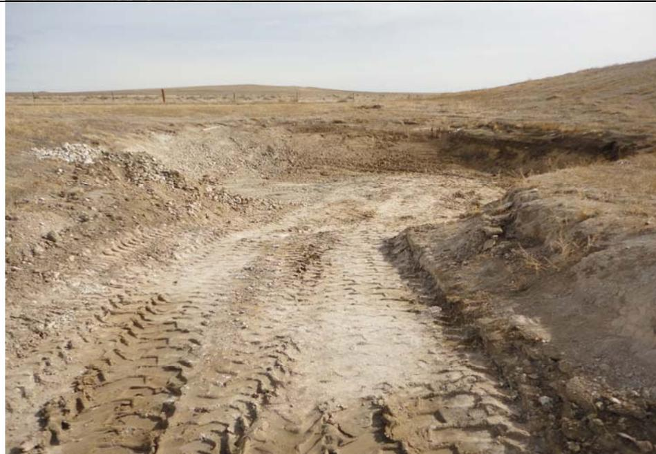
**Subject:** Photograph shows the detention pond on the east side of the Horsetail 19N pad following excavation. Confirmation soil sample HT19N-10 was collected from the base of the excavated detention pond.
