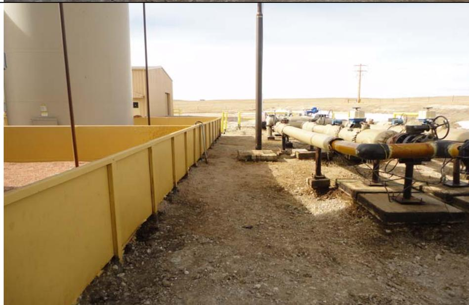
**Subject:** M&E Oilfield Services excavated impacted soil in the area of the spill using a skid steer and hand tools. Excavation activities were ongoing as of February 8, 2018. Confirmation soil sample, HT19N-6 was collected beneath the piping at the point of release to assess progress.
