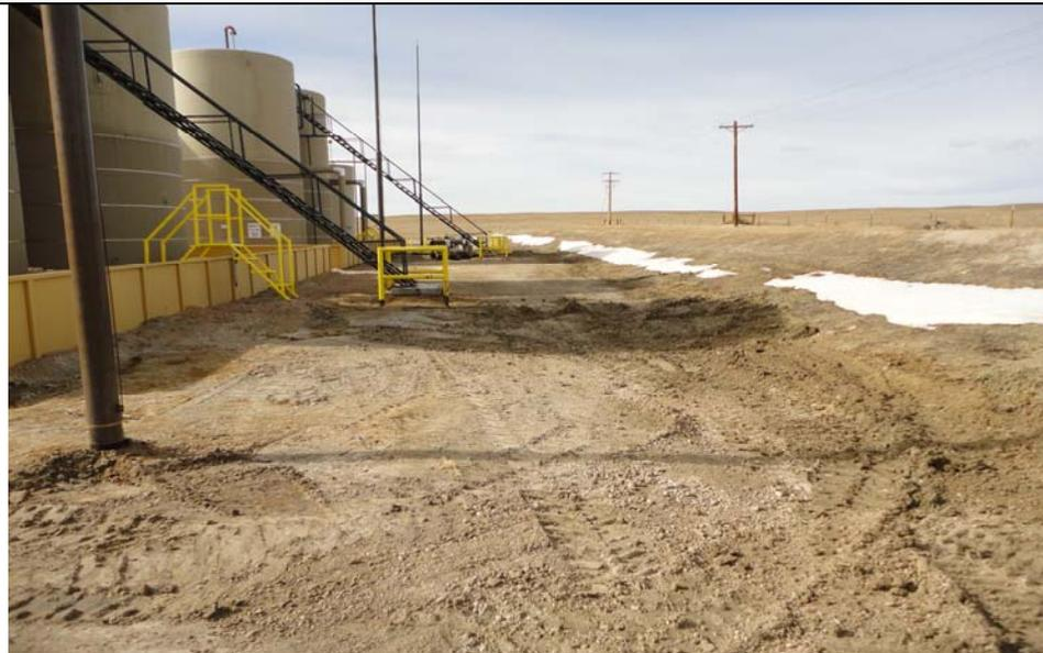
**Subject:** The produced water release extended along the north part of the Horsetail 19N pad and flowed east beyond the filtered produced water tank battery. Confirmation soil sample, HT19N-3 was collected near the northeast lightning rod shown on the left hand side of the photo. Confirmation soil sample HT19N-4 was collected near the base of the tank stairs.
