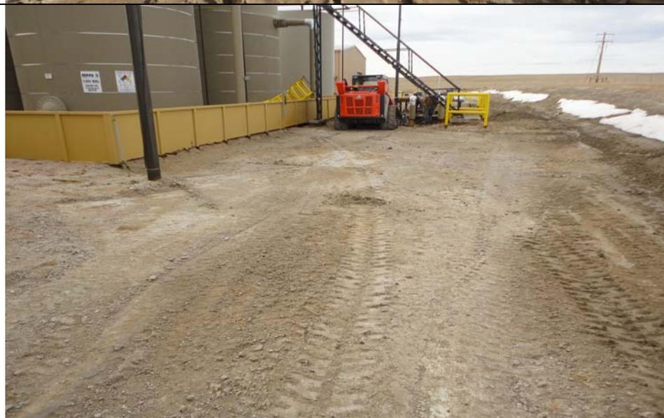
**Subject:** M & E Oilfield Services was retained to remove impacted soil at the site using a skid steer and hand tools. Excavation work was ongoing.
