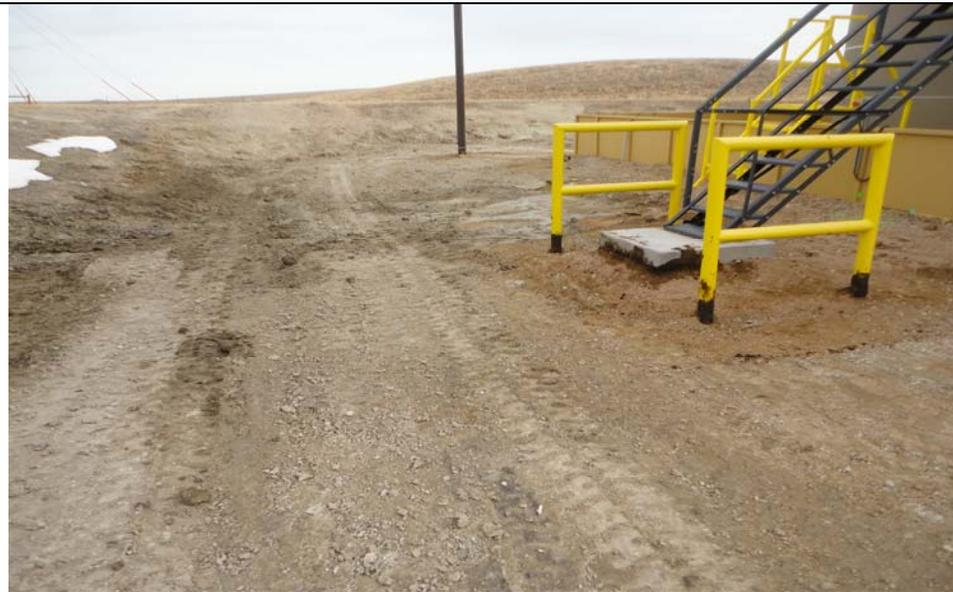
**Subject:** M&E Oilfield Services removed the impacted soils north and east of the filtered water tank battery using the skid steer. Olsson personnel collected confirmation soil sample HT19N-4 near the filtered produced water tank battery stairs.
