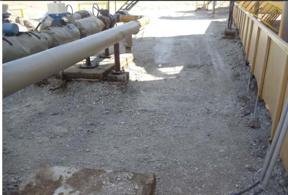
**Subject:** M&E performed additional excavation since the 02/08/2018 sampling event. Olsson collected confirmation soil samples near locations where previous soil samples had total petroleum hydrocarbons (TPH) as diesel range organics (DRO) above the COGCC Table 910-1 standard of 500 mg/kg.
