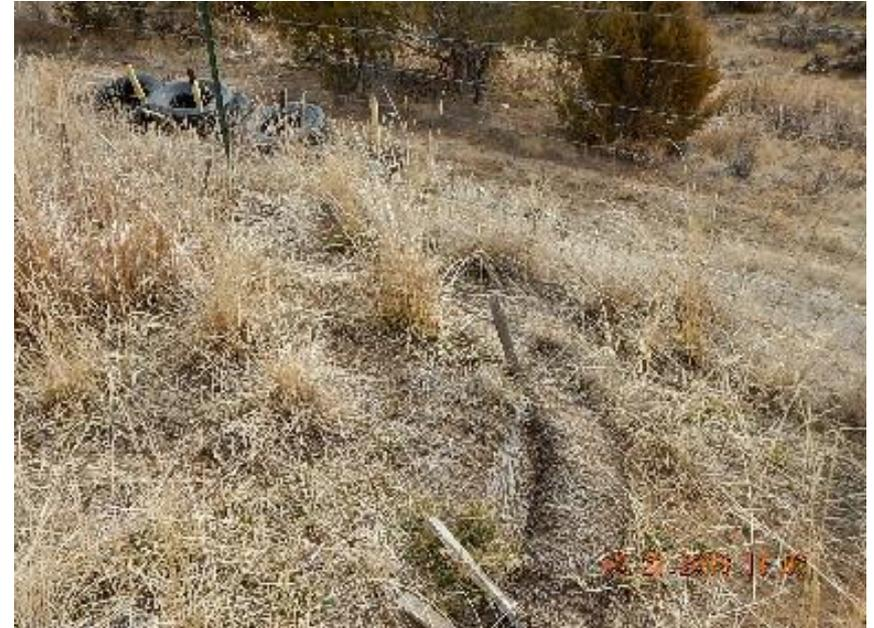
Photo 4: Deteriorated waddles along E perimeter fencing.
