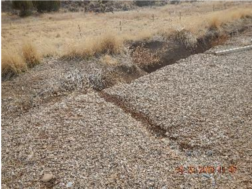
Photo 3: Erosion channel on S edge of disturbed area feeding stormwater into gulley.
