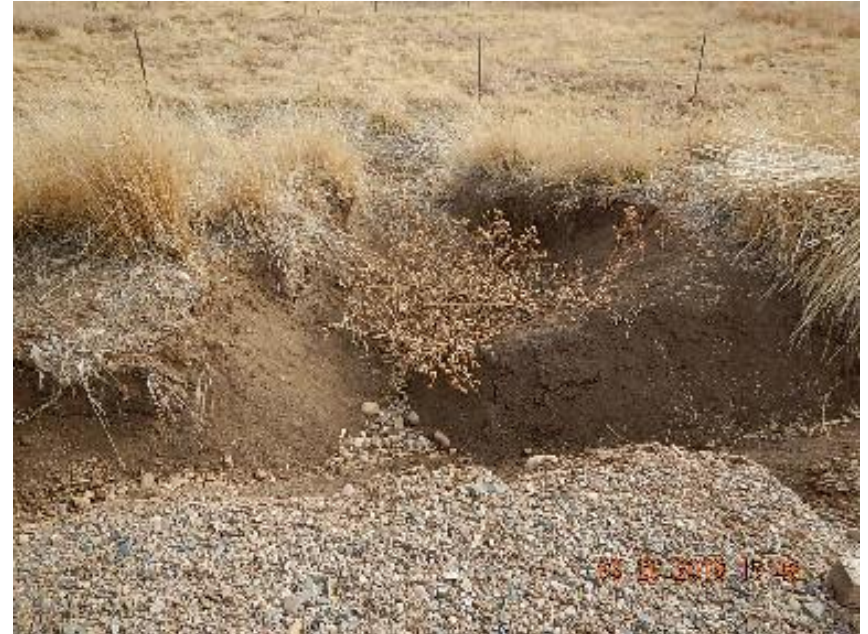
Photo 4: Erosion gulley on S perimeter of location.
