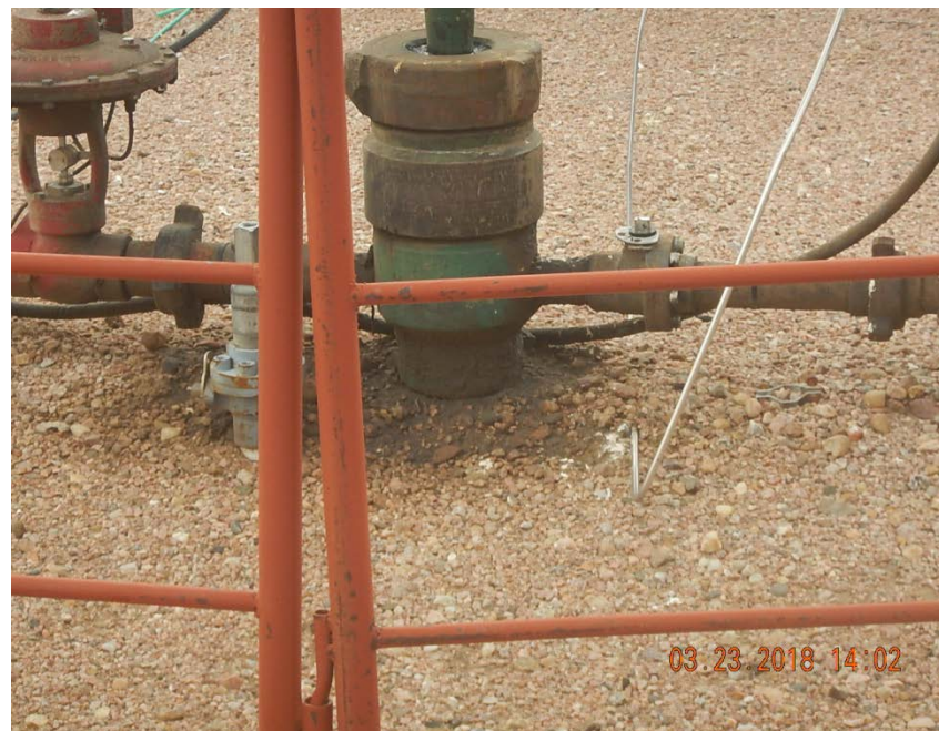
Photo 2: Stained soil at wellhead
