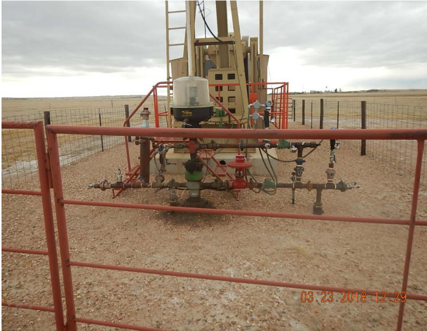
Photo 1: Wellhead, looking S
