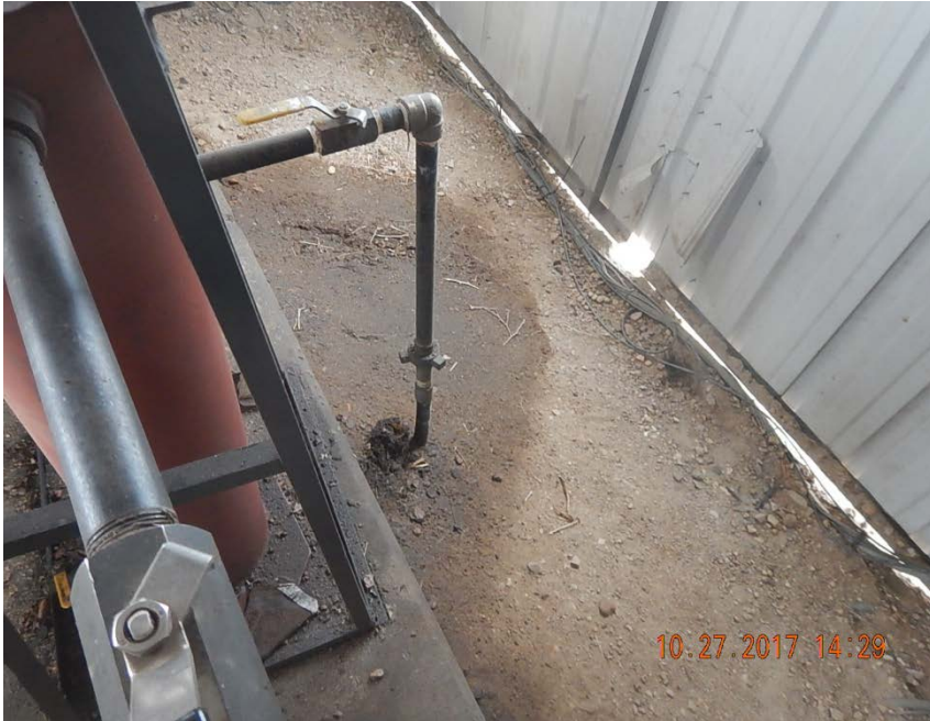
Photo from prior inspection for comparison
