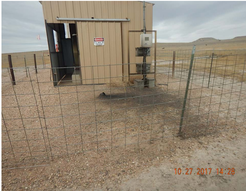
Photo from prior inspection for comparison
