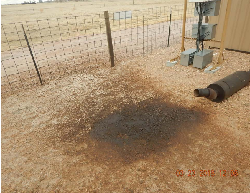
Photo 3: Stained soil at exhaust
