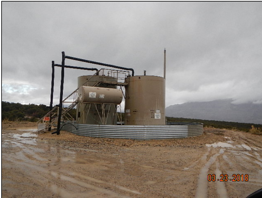
Photo 1. Repaired tank containment.
