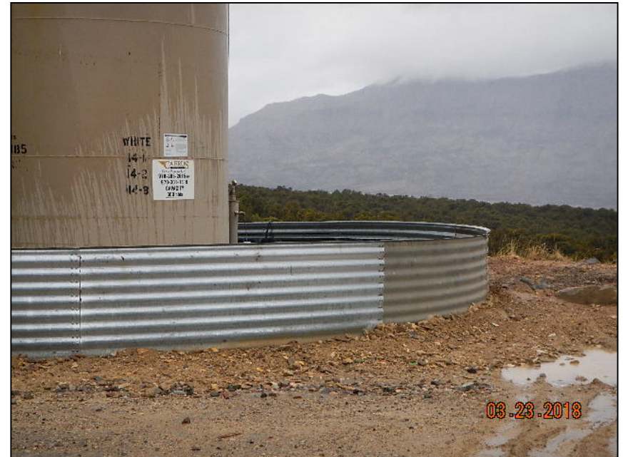
Photo 2. Repaired tank containment.
