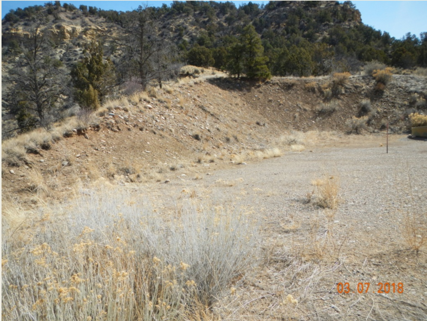
Photo 4. View of the northern portion of the project area from the northwestern corner facing eastward. Steep cut-slope supports sparse revegetation. This needs to be monitored and further slope stabilization measures taken if noticeable erosion is occurring.
