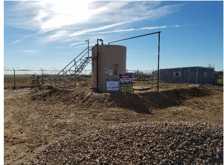
Photo 2. Tank battery
