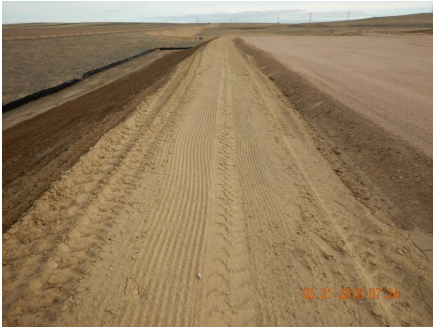
Photo 7. Photo taken from the western location, facing North. Operator has installed a moat system around the well pad perimeter. Fill and cut slopes have been seeded.
