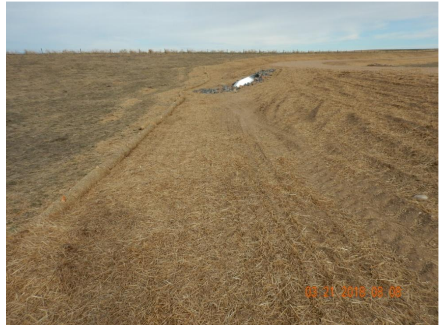
Photo 4. Photo taken from a portion of the access road, facing North. Operator has installed culverts with a stabilized outlet in conjunction to the roadside ditch, installed straw wattles, straw mulched and seeded the roadside ditch.
