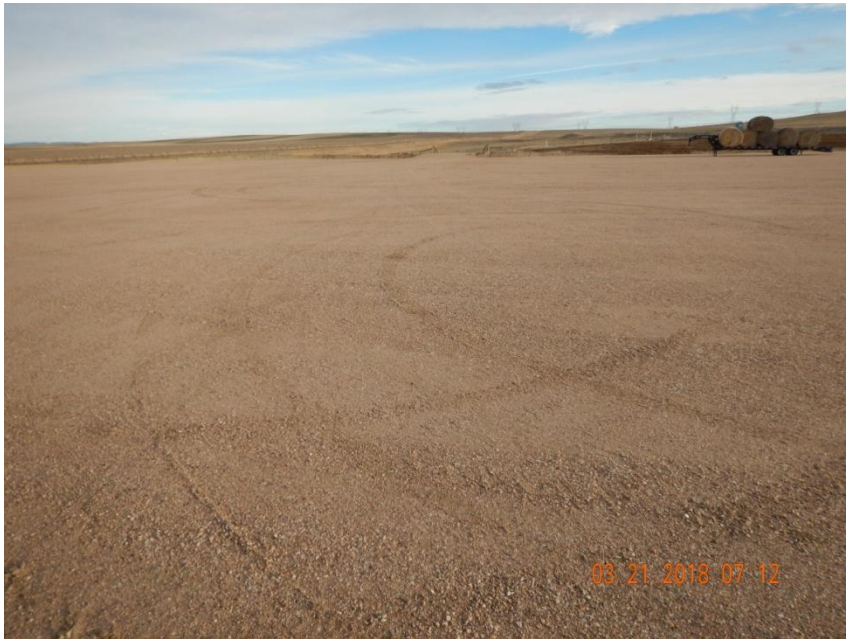
Photo 5. Photo taken from the approximate center of location, facing Northeast. Operator has installed and compacted gravel throughout the location.
