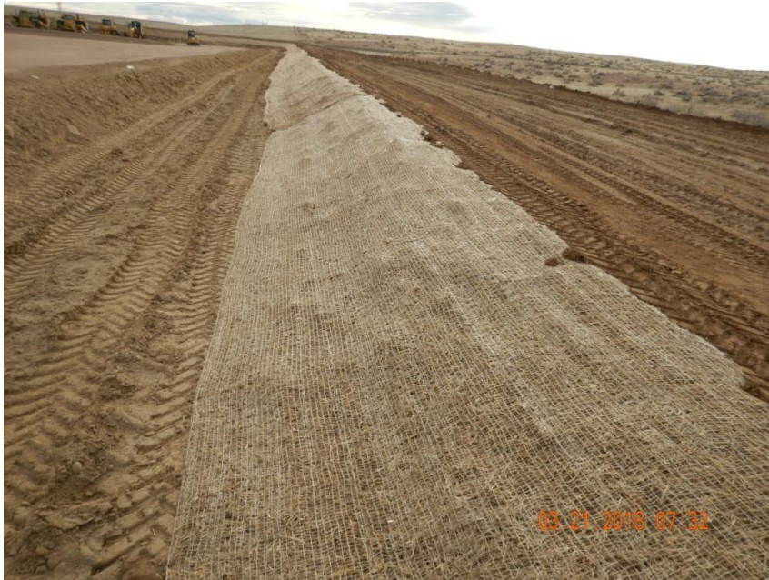
Photo 9. Photo taken from the southern location on the topsoil stockpile, facing East. Operator has seeded portions of the topsoil stockpile for long-term stabilization and protection of topsoil, and installed erosion control blankets along the fill slope of the topsoil stockpile.
