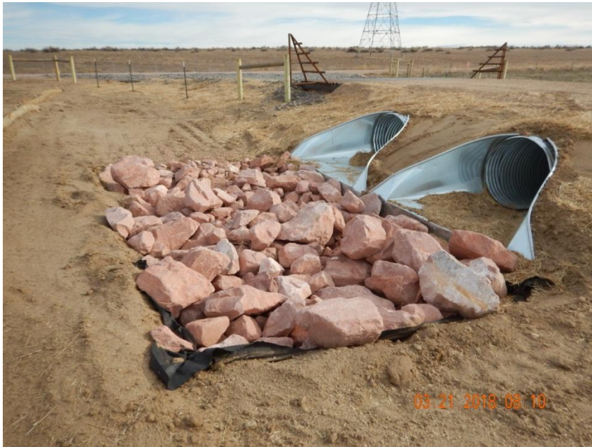
Photo 3. Photo taken from the location entrance, facing North. Operator has installed culverts with a stabilized outlet in conjunction to the roadside ditch.
