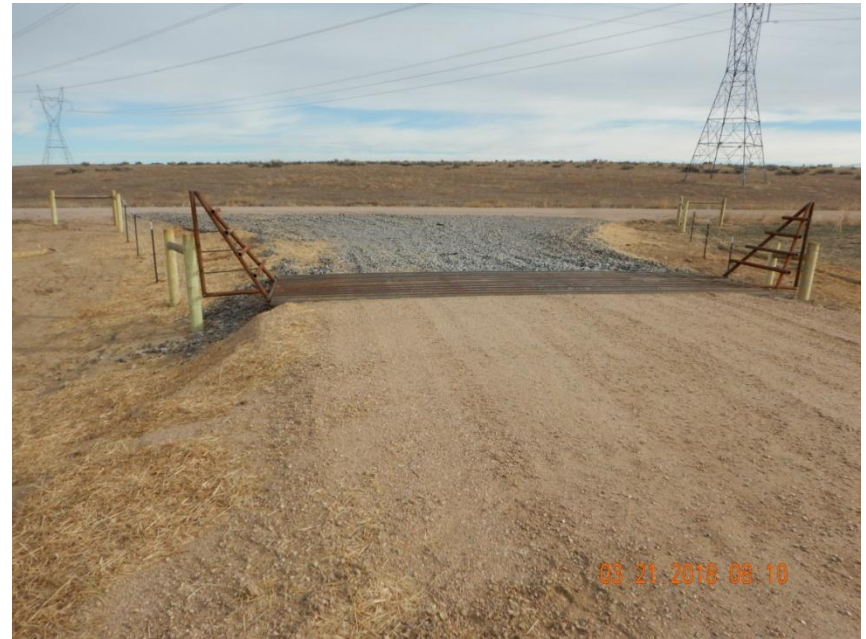
Photo 2. Photo taken from the location entrance, facing North. Operator has installed a vehicle tracking device and appears to be in proper functioning condition.
