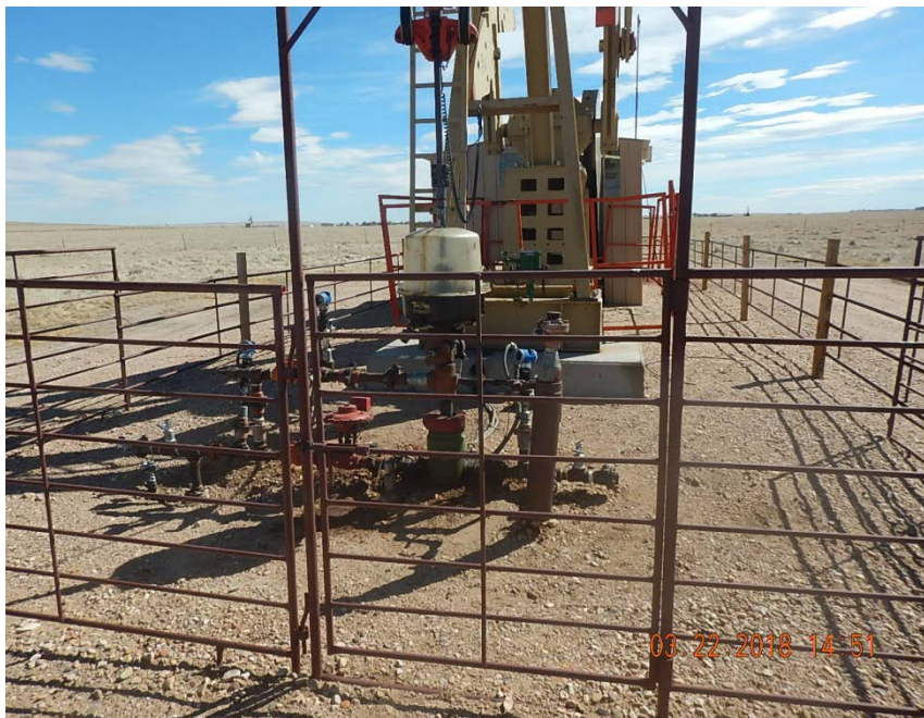
Photo 1: Wellhead, looking S
