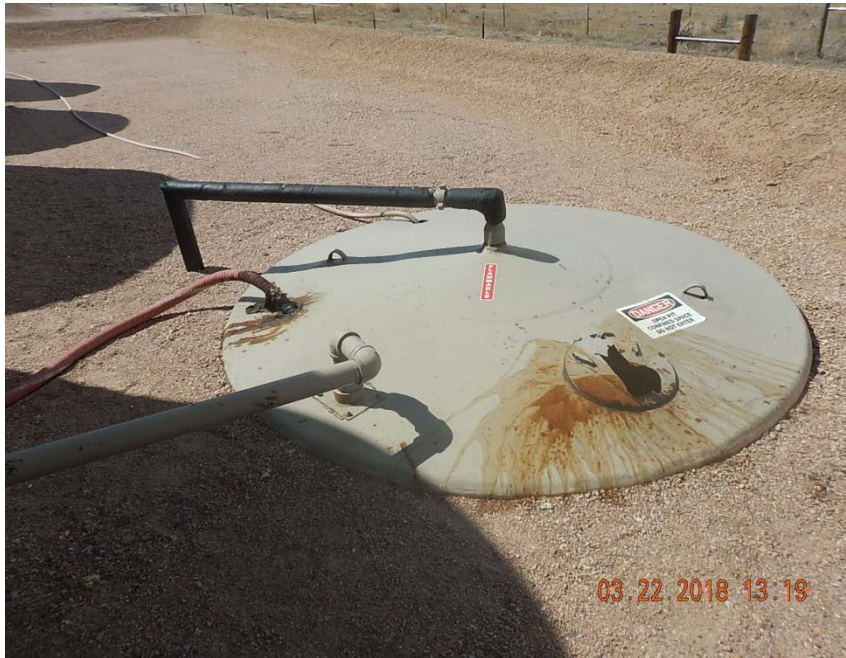
Photo 3: Tank is open to wildlife entrance, stained soil around tank.
