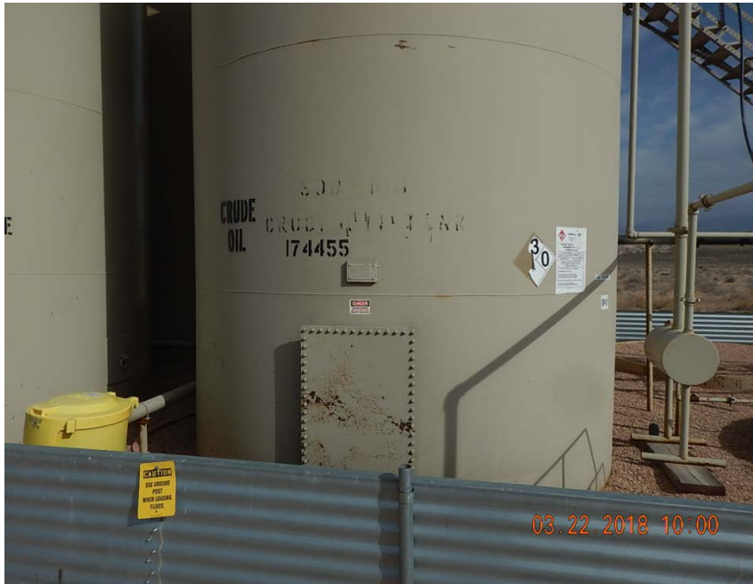
Photo 3: Damaged NFPA decals
