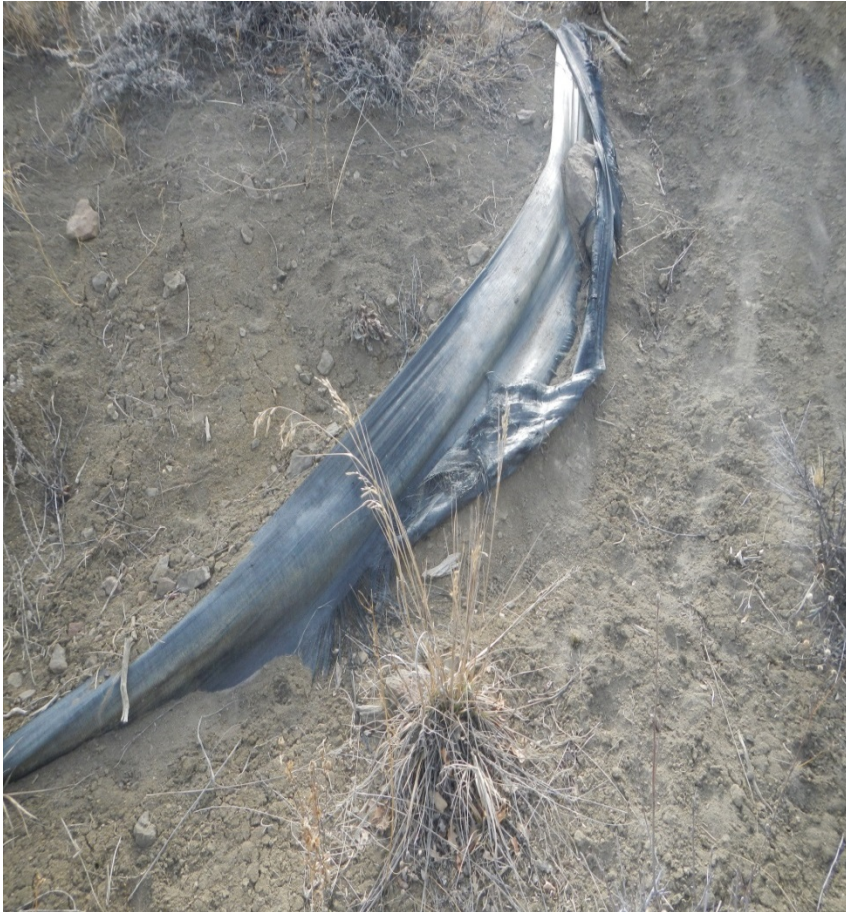
Photo#5: Detail of silt fence debris along base of fill slope.
