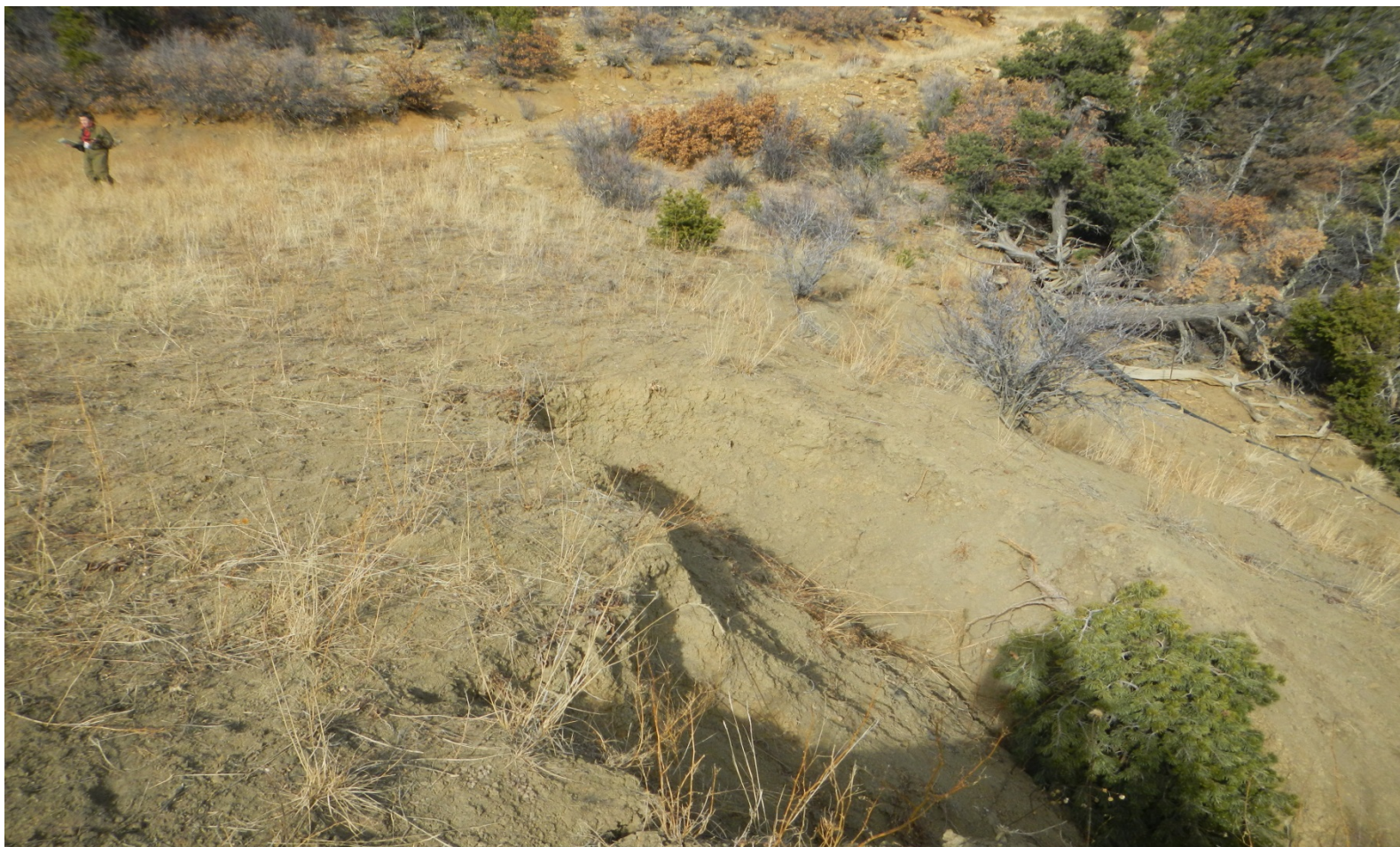
Photo#2: View Northeast along severely eroded fill slope.
