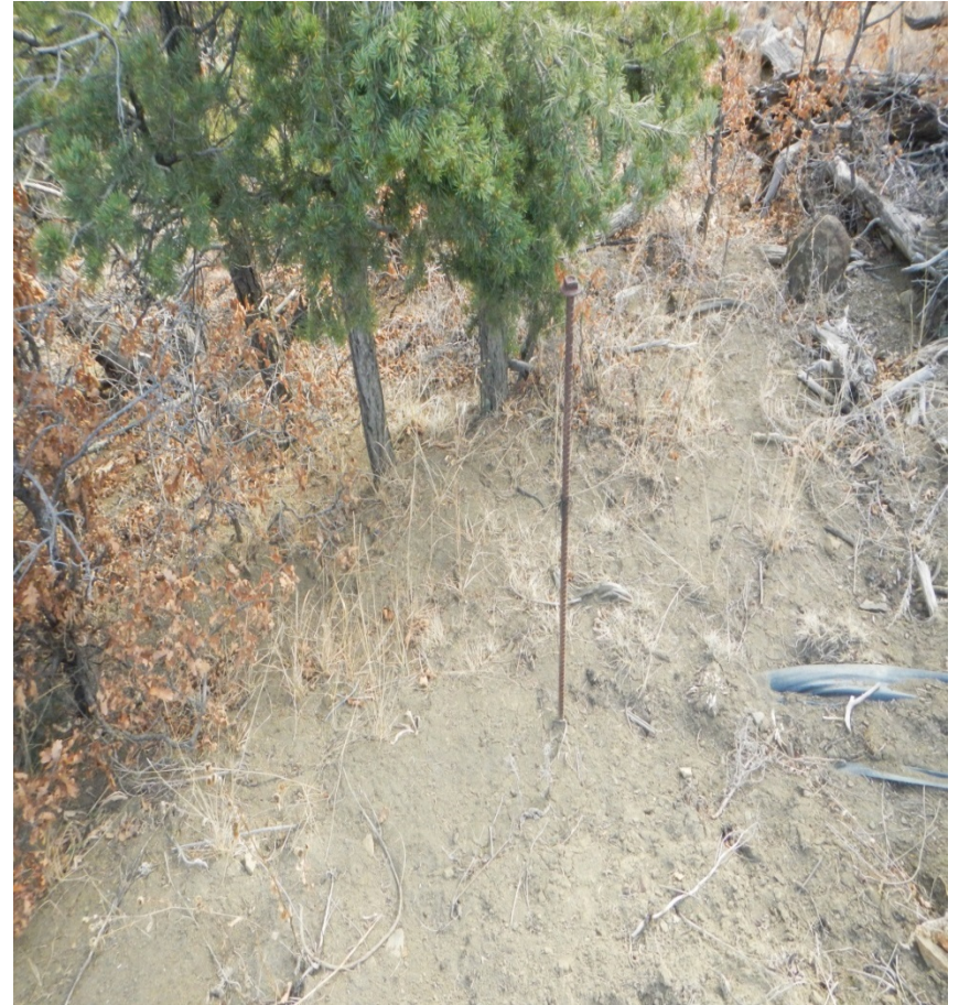
Photo#6: Roof anchors, used as silt fence support still in place at base of fill slope.
