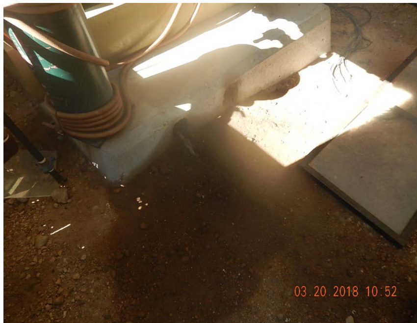
Photo 3: Stained soil, residue at engine
