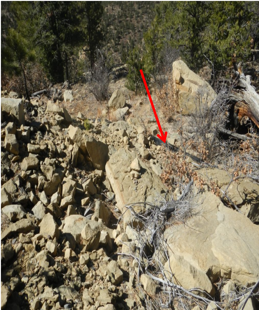
Photo#5: Silt fence at base of fill slope has become debris. Arrows indicate silt fence position
