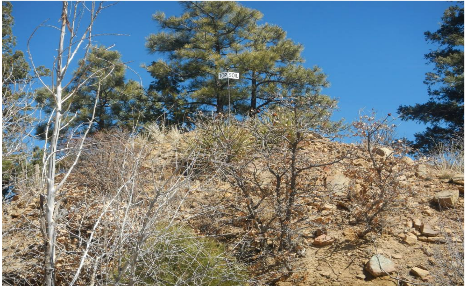
Photo#4: Sign at top of cut slope indicating unutilized top soil stockpile.
