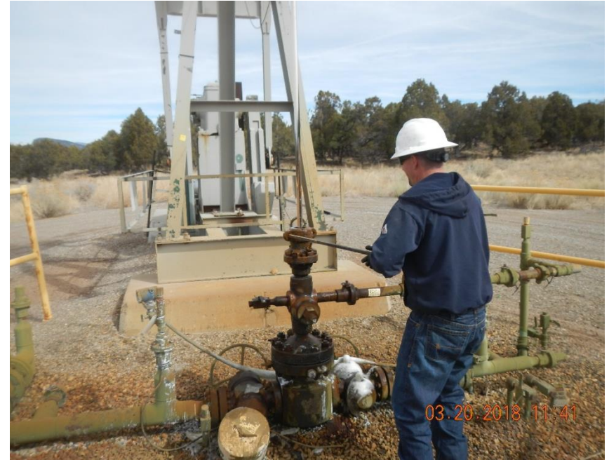
Hilcorp representative replacing well head packing.
