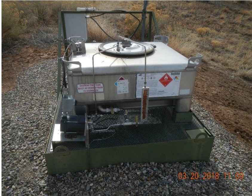
Chemical injection system on secondary containment.
