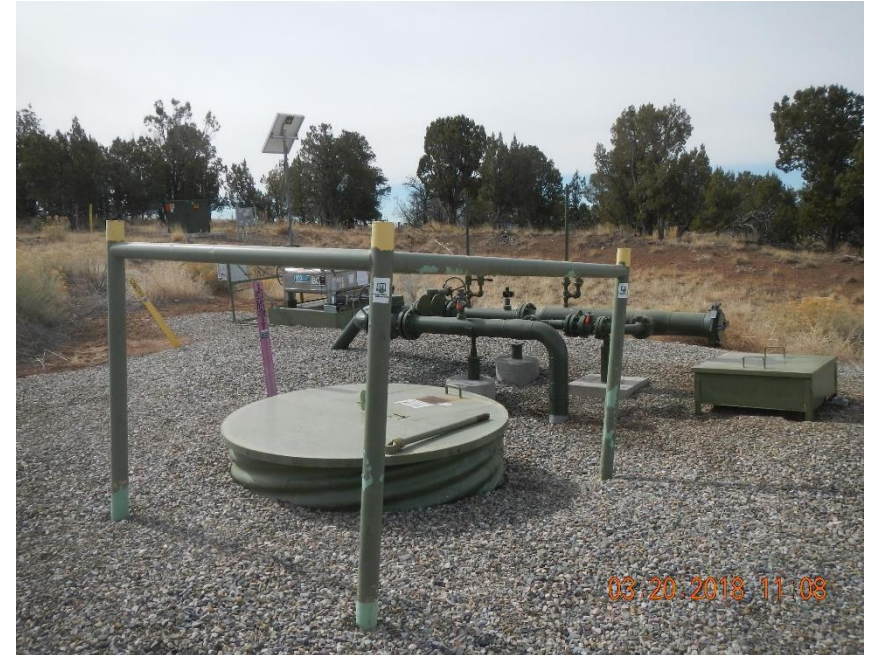
Below grade valve access and pig launcher.
