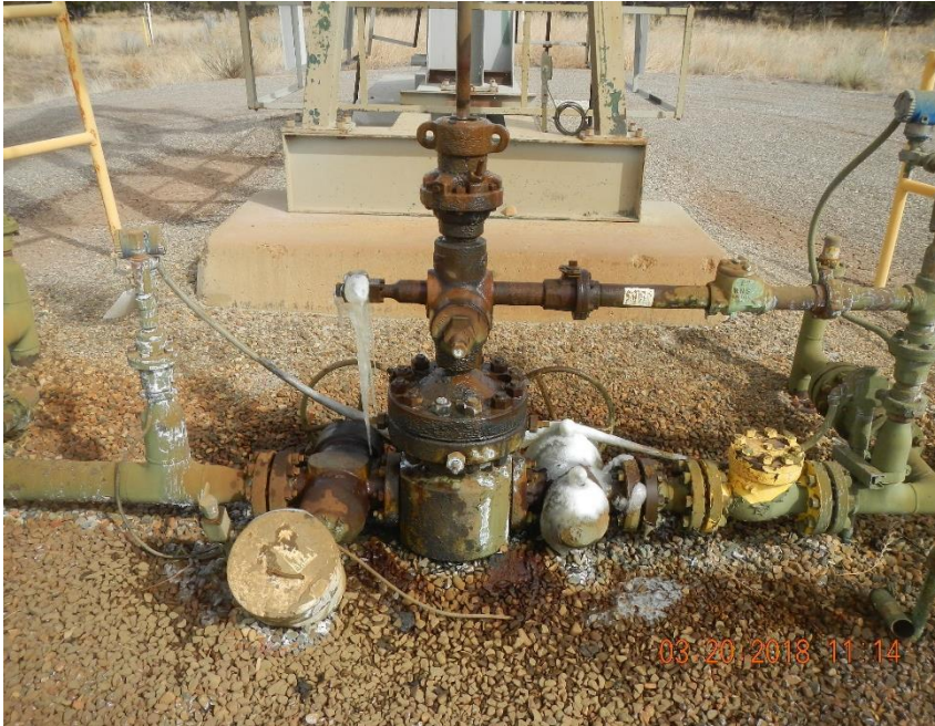
Well head packing was leaking during this field inspection. Ice had formed on well head and production piping.
