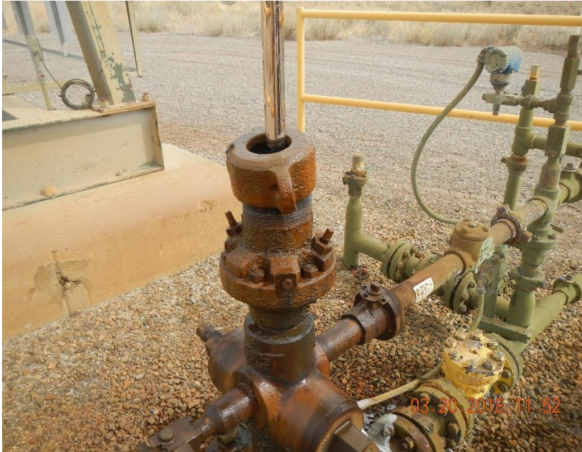
Compression fitting removed to replace packing.
