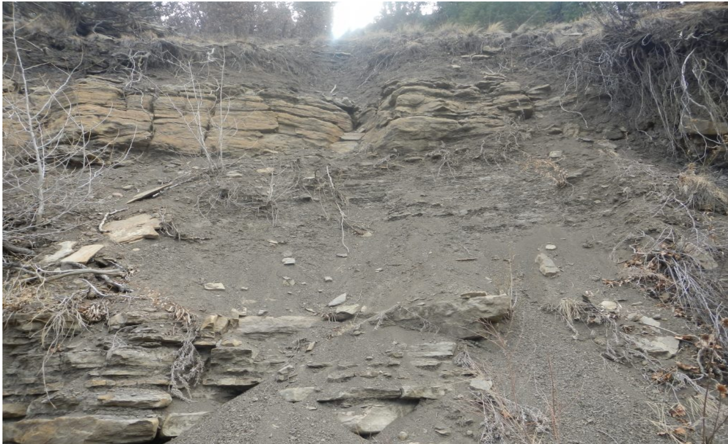
Photo#2: Unstable conditions of East Cut Bank of Access Rd.
