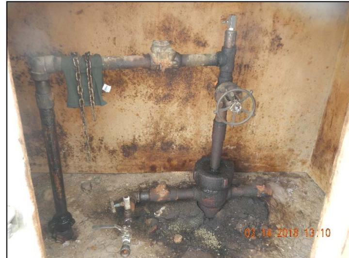
**Photo 2. Stained soil at wellhead.**
