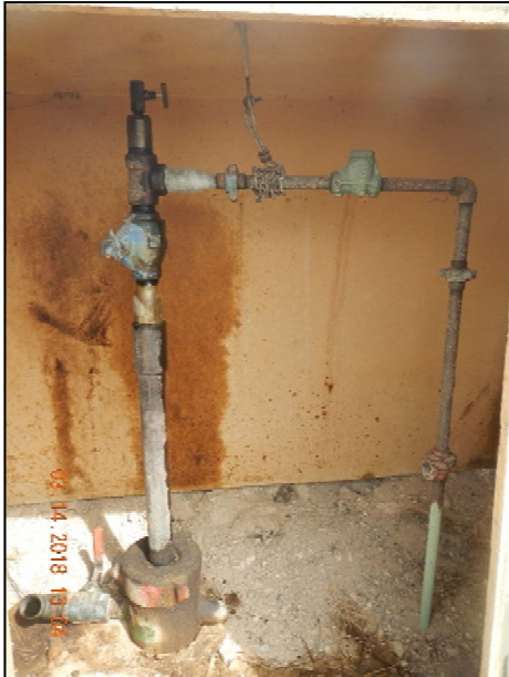
Photo 2. Stained soil and fluid in tubing.
