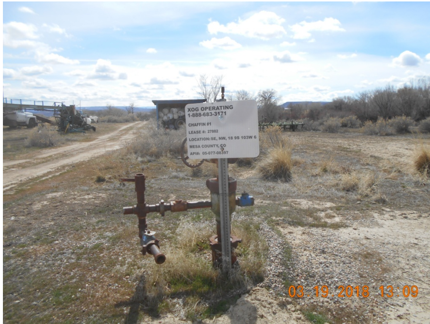
Wellhead with sign
