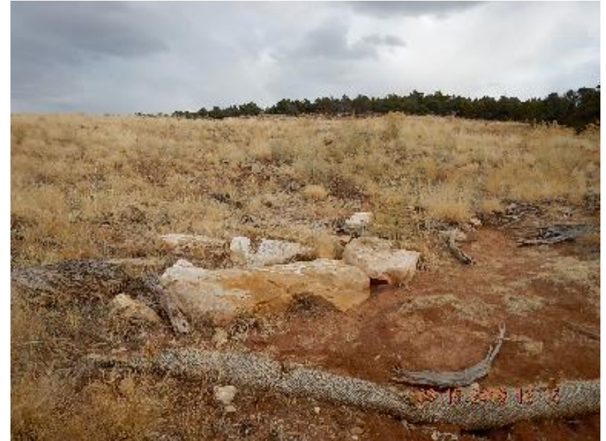
Photo 6: Natural rock and waddle check dam and sediment trap.
