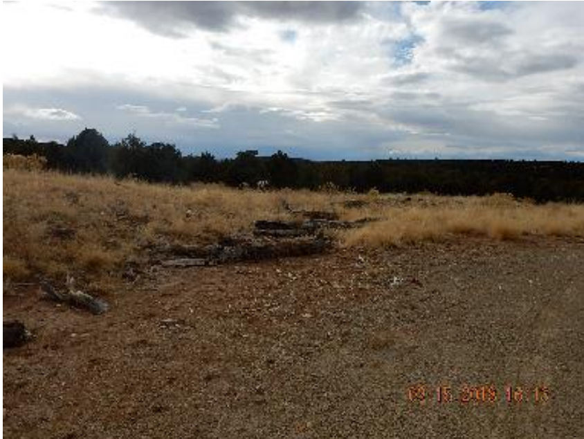
Photo 5: Use of natural materials as check dams and sediment traps.
