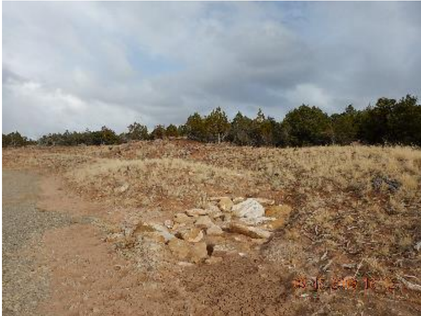
Photo 3: Natural rock check dam and rip rap.
