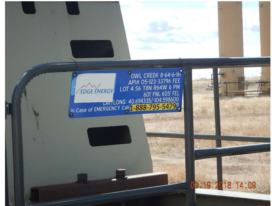
Photo 4: Wellhead sign has decal for current operator. Emergency number is for prior operator.
