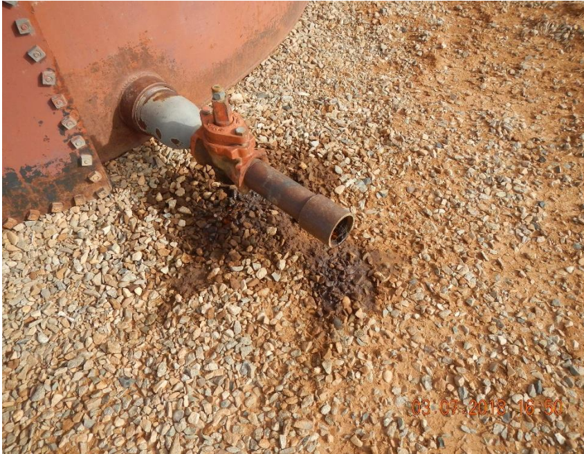
Additional valve on western tank with stained soil.
