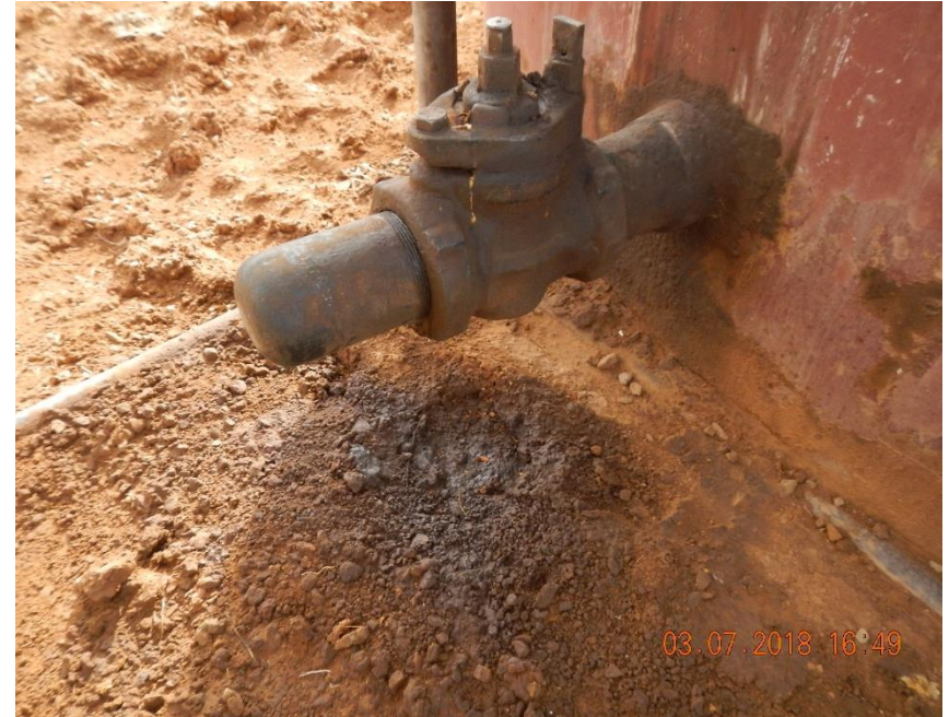
Stained soil beneath load out valve on western tank.
