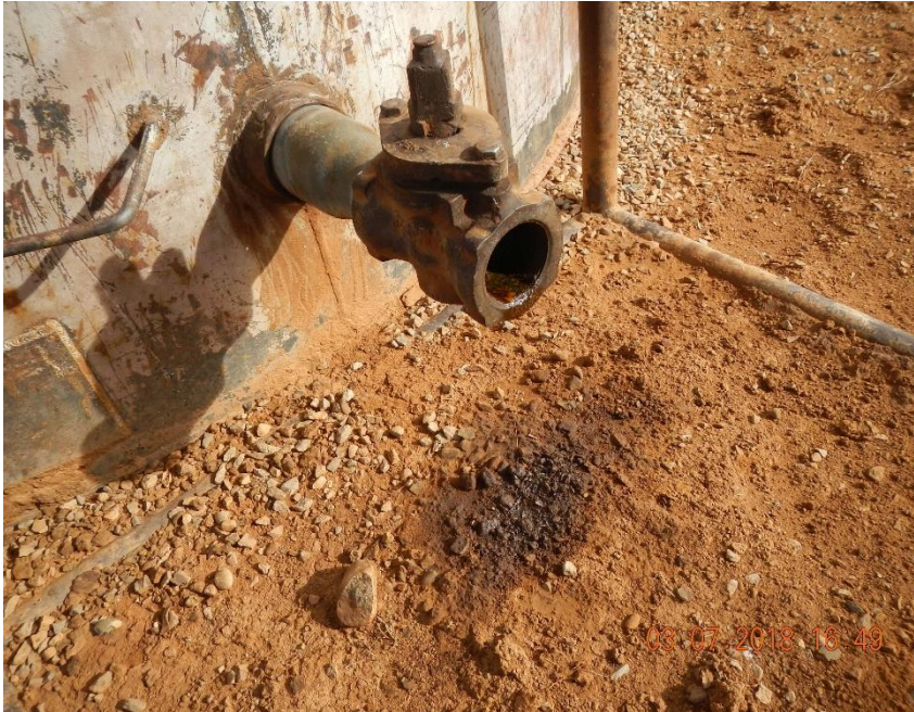
Stained soil beneath load out valve on eastern tank.
