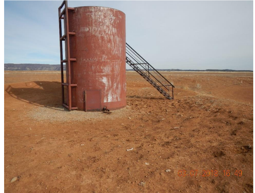
Inadequate secondary containment berm capacity.
