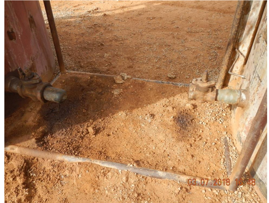
Stained soil beneath tank load out valves.
