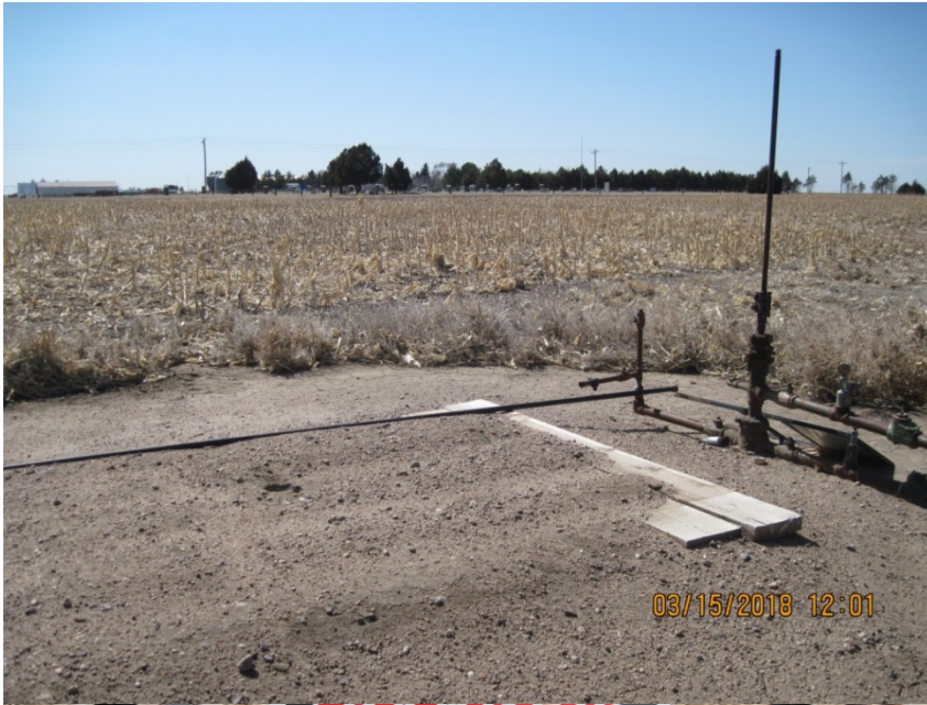
3. Wellhead equipment has been removed
