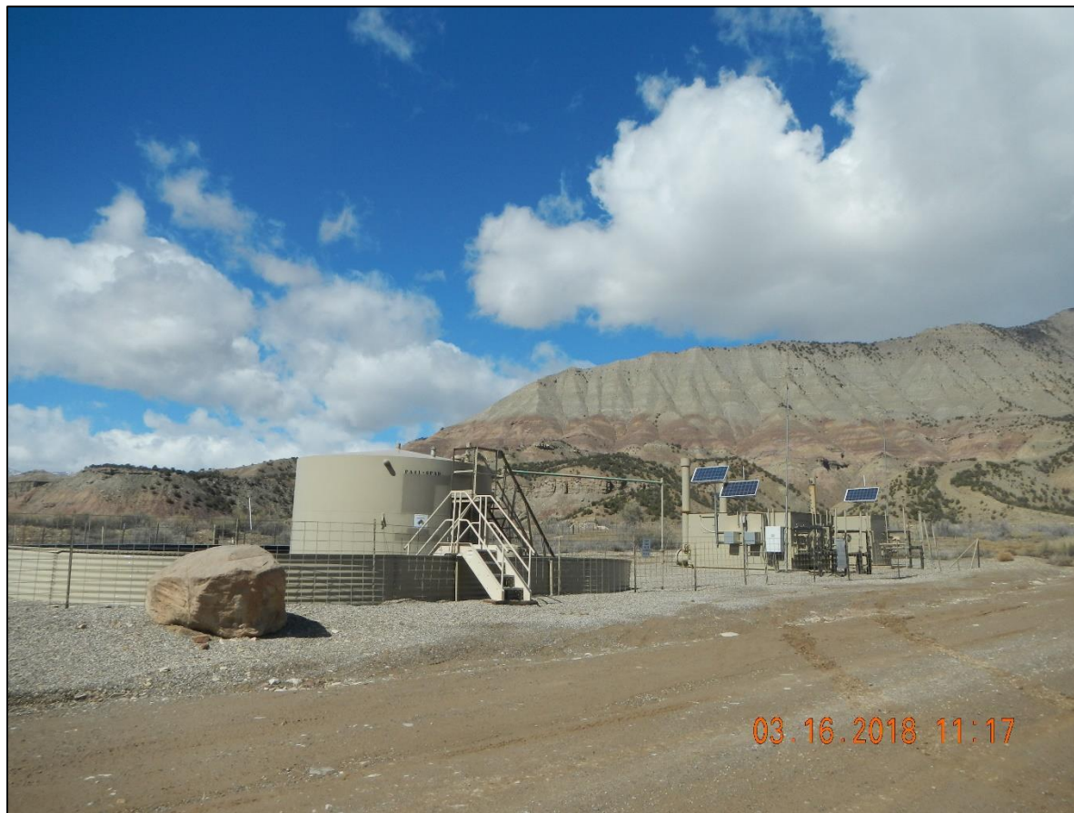
Tank battery and separators.
