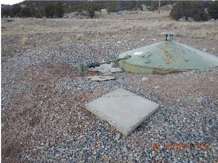
Photo 5: Concrete base and pipe insulation wraps beside produced water tank.
