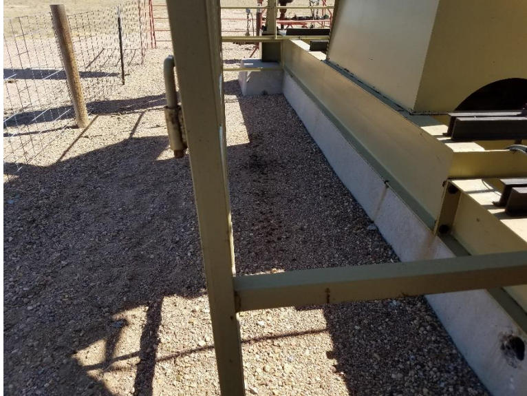
Photo 3. stained soil under pumpjack weights
