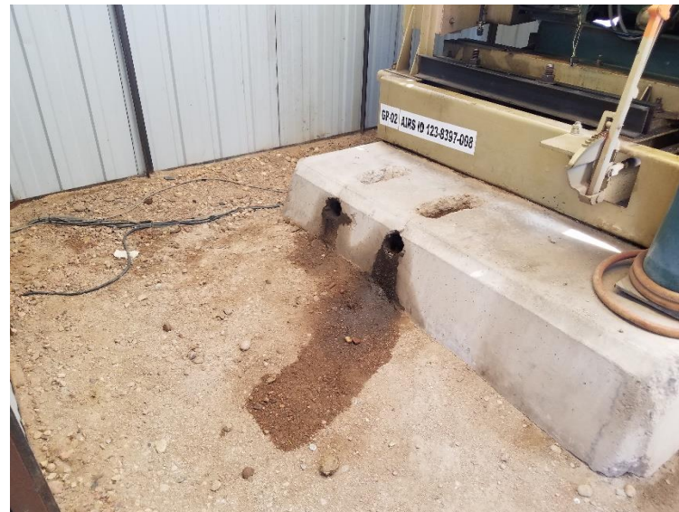
Photo 2. stained soil in motor room
