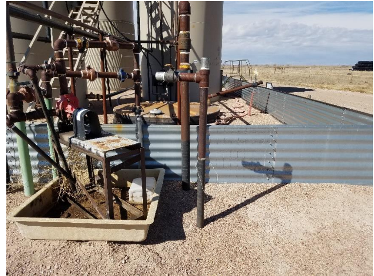
Photo 2. unmarked riser east of battery berm
