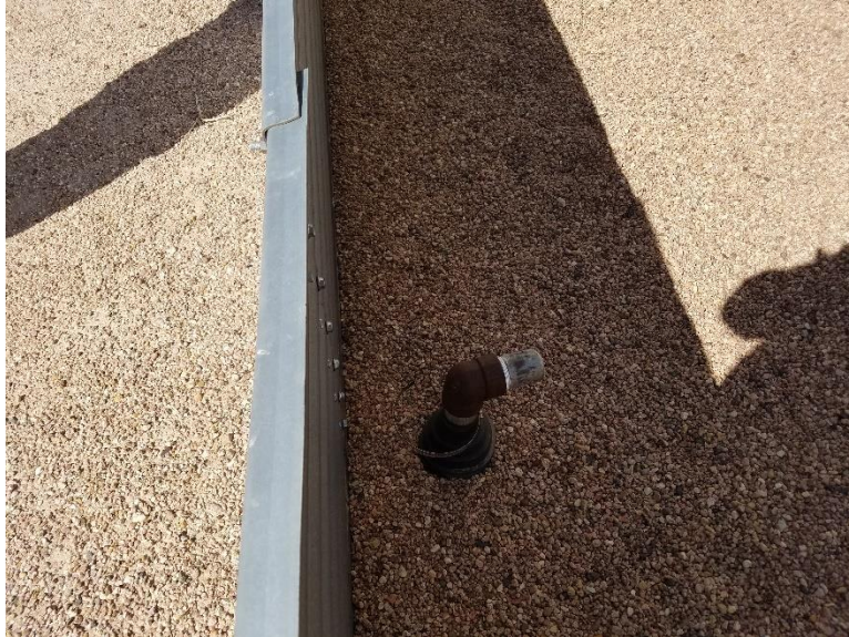
Photo 3. unmarked riser inside berm on south side
