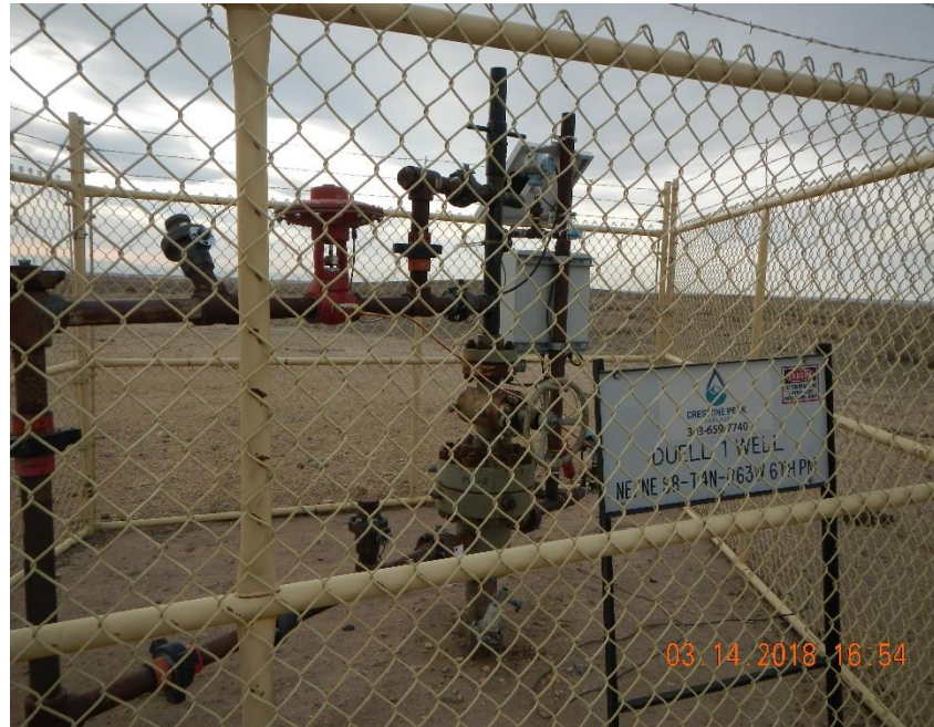
Wellhead from SE view
