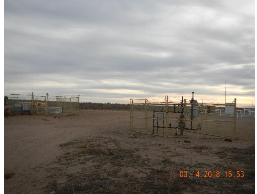
Site location from NW view
