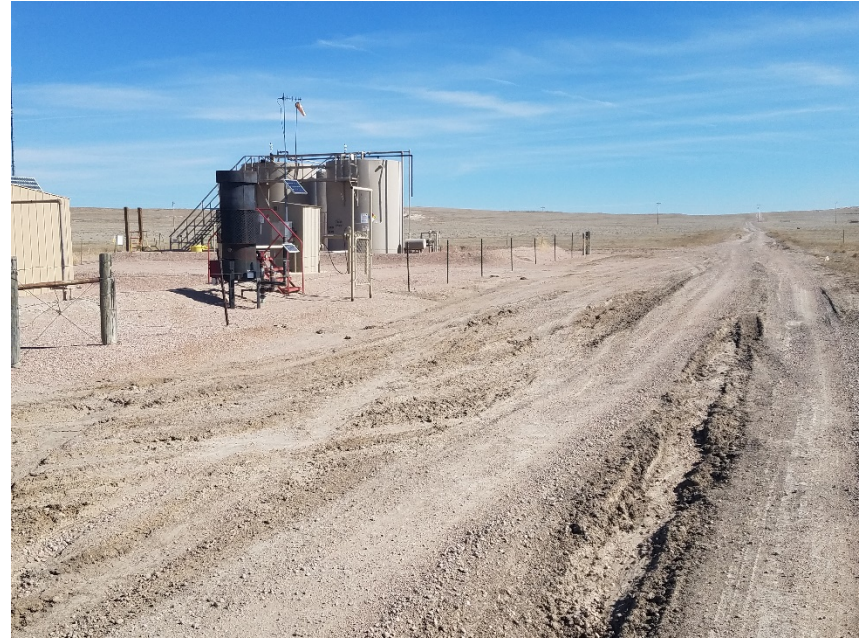
Photo 8: Stormwater erosion on S. side of location
