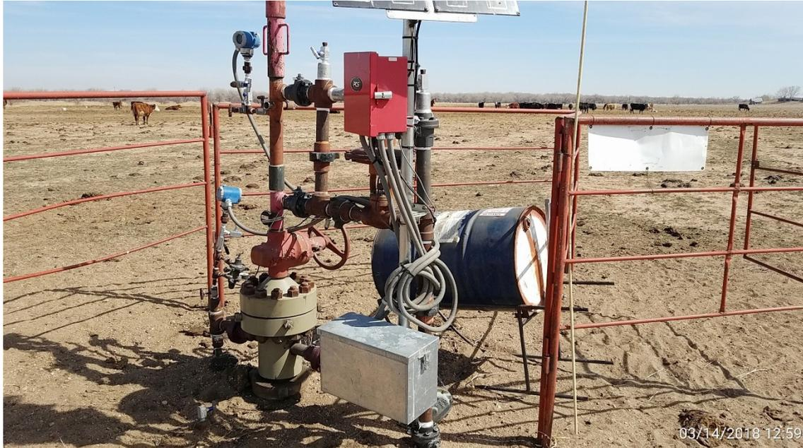
**Wellhead. Corrective action: Unused equipment (Methanol barrel & pump). Remove to comply with rule 603.f**
