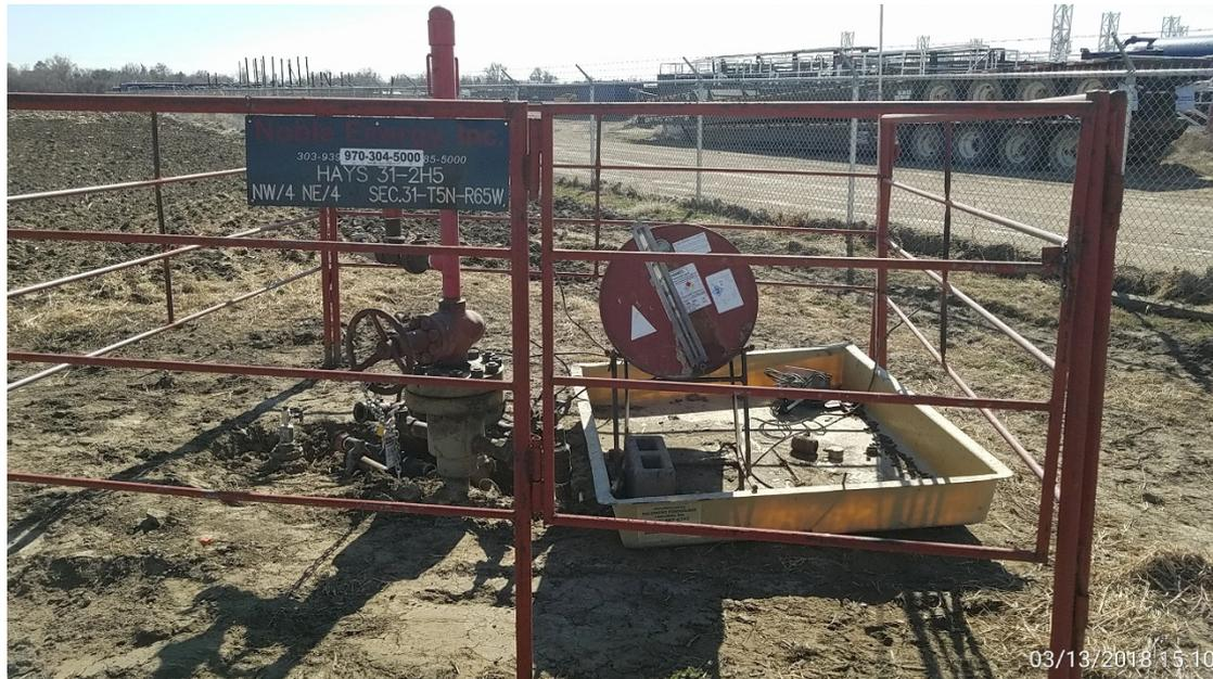
**Wellhead. Corrective Action: Remove unused equipment per rule 60.f (Methanol barrel, pump, & containment)**
