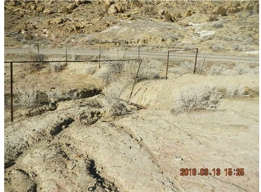
Weeds/Brush/Erosion cuts in blow down pit
