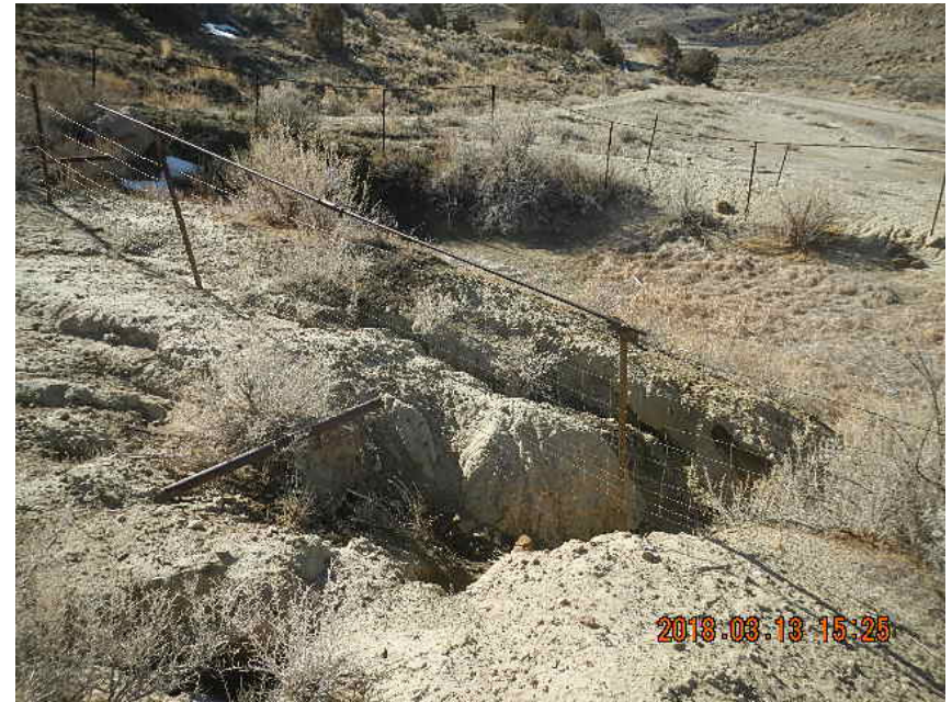
Weeds/Brush/Erosion cuts in blow down pit
