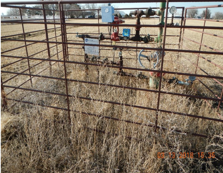
Wellhead with weeds from SE view. Sign needs PDC contact information.
