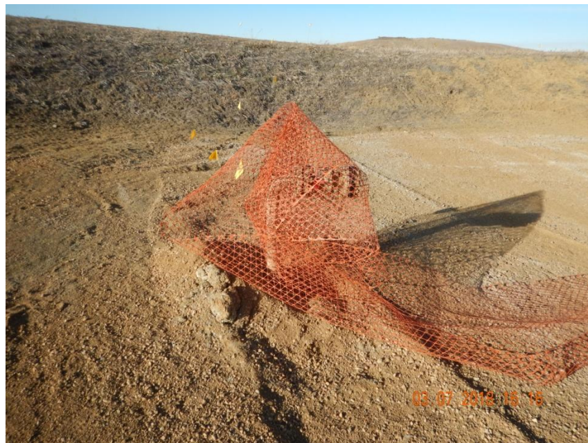
Photo 8. Close-up photo taken of the abandoned riser. Riser was locked out/tagged out with an Extraction contact.
