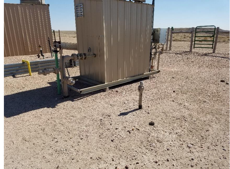
Photo 12. unmarked riser
