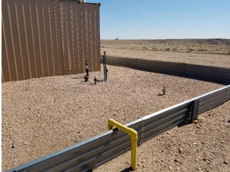
Photo 13. unmarked risers
