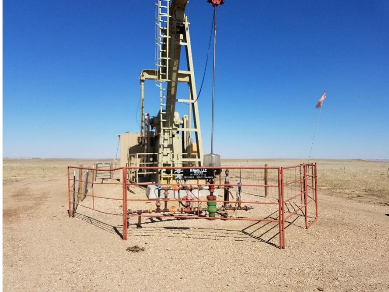
Photo 1. Signs at wellhead
