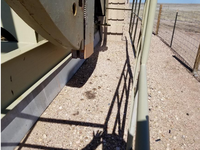
Photo 1. Stained soil under pumpjack
