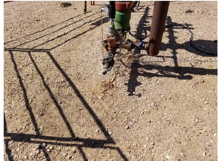
Photo 2. stained soil around wellhead
