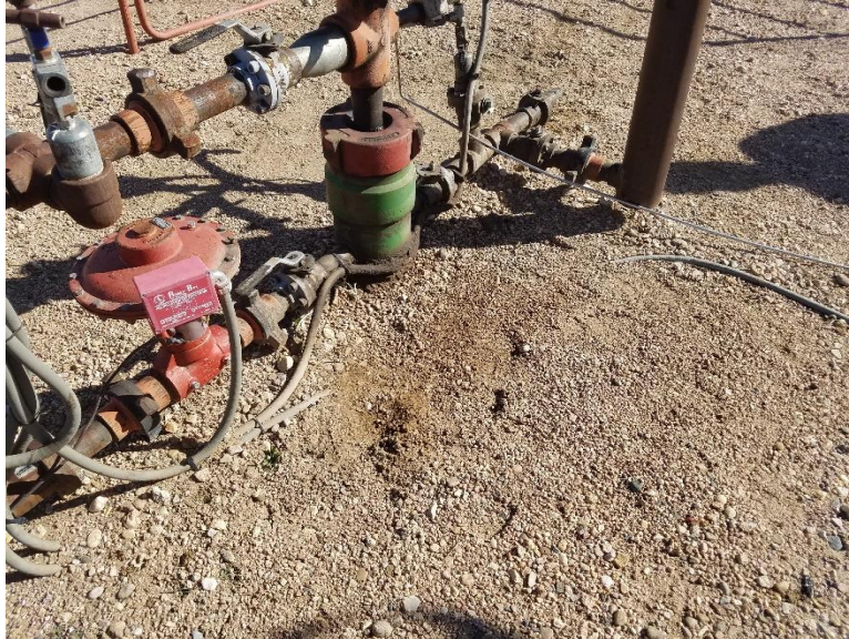
Photo 3. stained soil at wellhead
