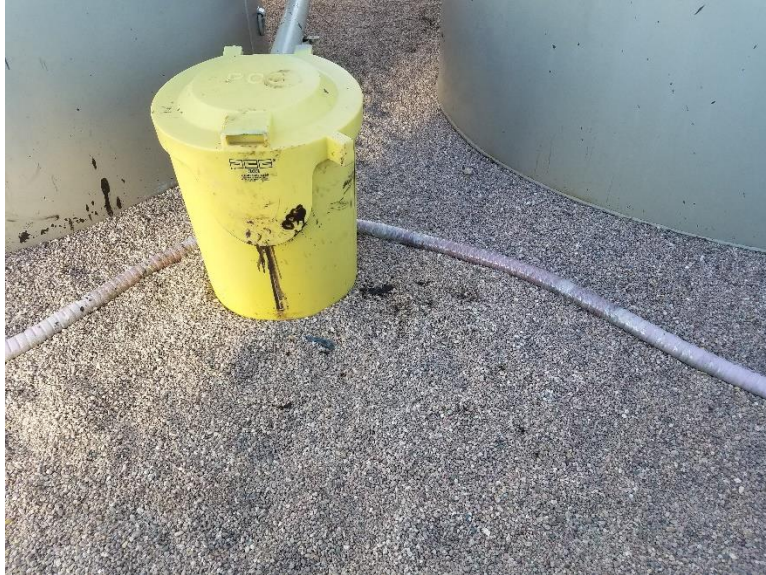
Photo 7. stained soil near load out
