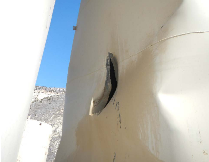
Impact damage to decommissioned AST
