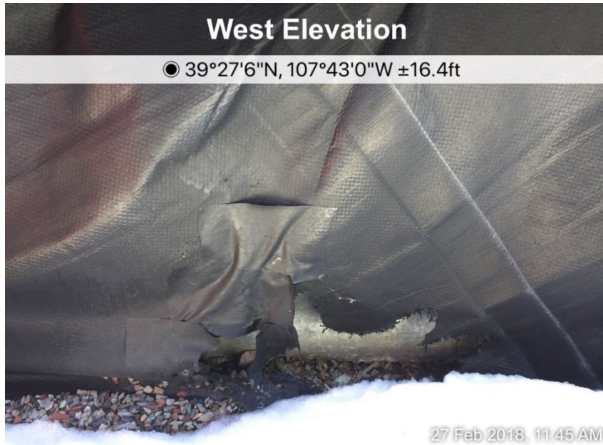
Photo # 1 Hole in Tank Containment
