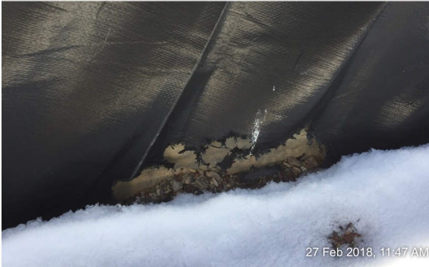
Photo #3 Hole in Tank Containment
