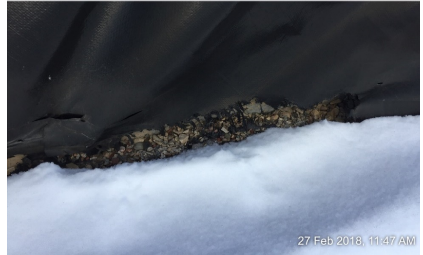
Photo #4 Hole in Tank Containment
