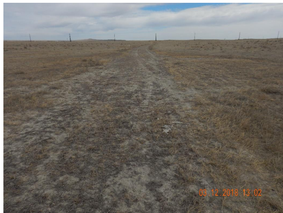
Photo 4: Photo taken from the access road, facing east. Germination and vegetative establishment is evident, however reclamation on the road does not appear to be progressing and supplemental reclamation will likely be required.
