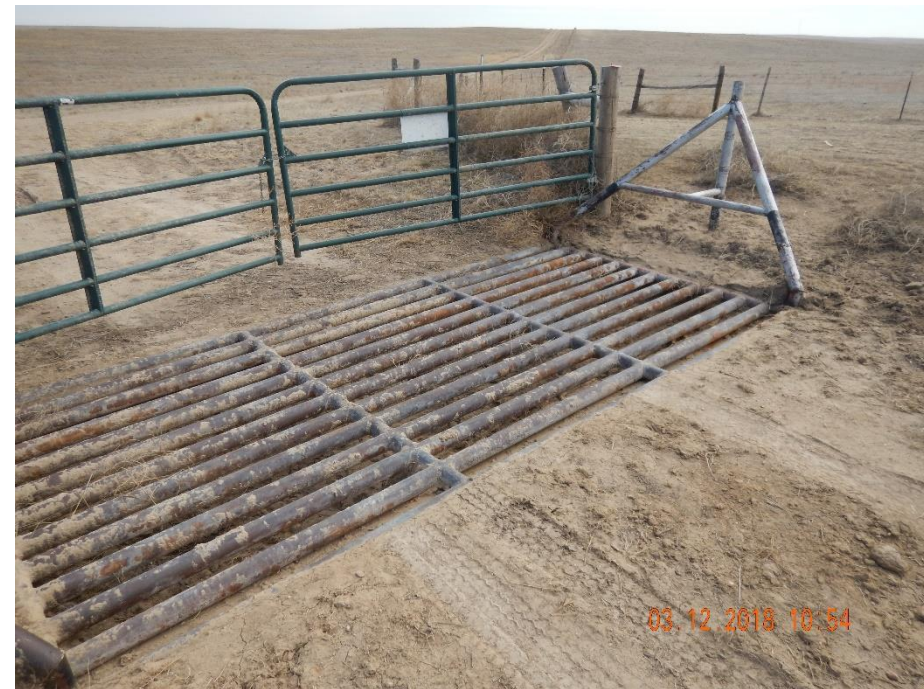
Photo 4: Photo taken from the access road. Photo shows cattle guard has not been removed, though maintenance appears to have been conducted. Sundry #401502788, operator states “surface owner does not want BMP removed and is in the process of filing paperwork to accommodate request”. At time of inspection, no variance has been submitted, location will remain out of compliance until variance request has been approved or BMP removed per CA
