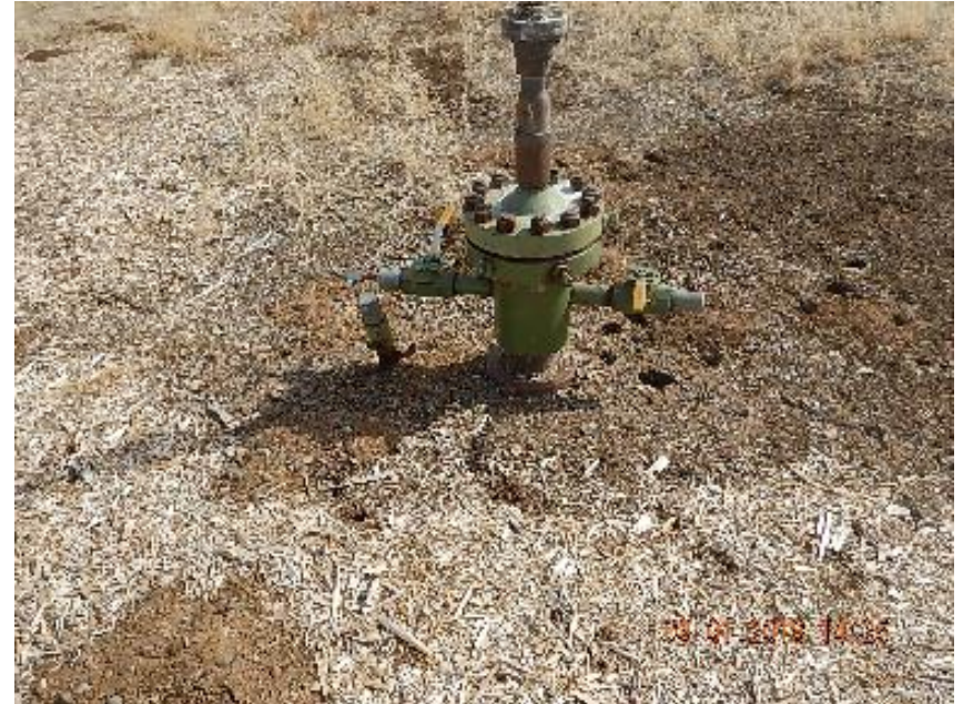
Photo 4: Debris removed from wellhead area.
