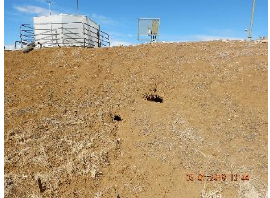
Photo 4: Animal burrow on S fill slope below sink hole.
