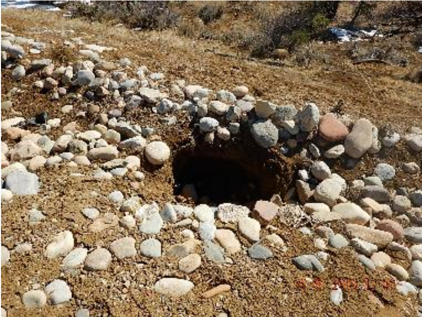
Photo 3: Sink hole at top of S slope.
