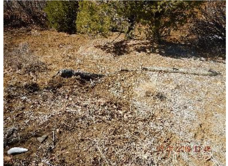
Photo 6: Waddle used as check dam that is full on backside.
