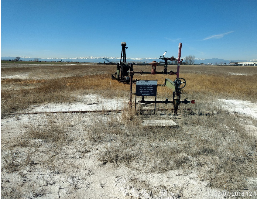
Wellhead, Corrective actions: Control weeds at wellhead and lease road. Remove unused equipment (Flow iron & pumping unit).
