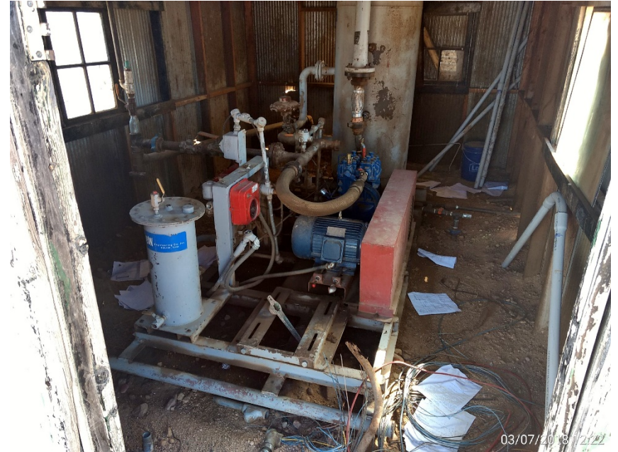
Sales Compressor Detail, Corrective action: remove trash from housing.
