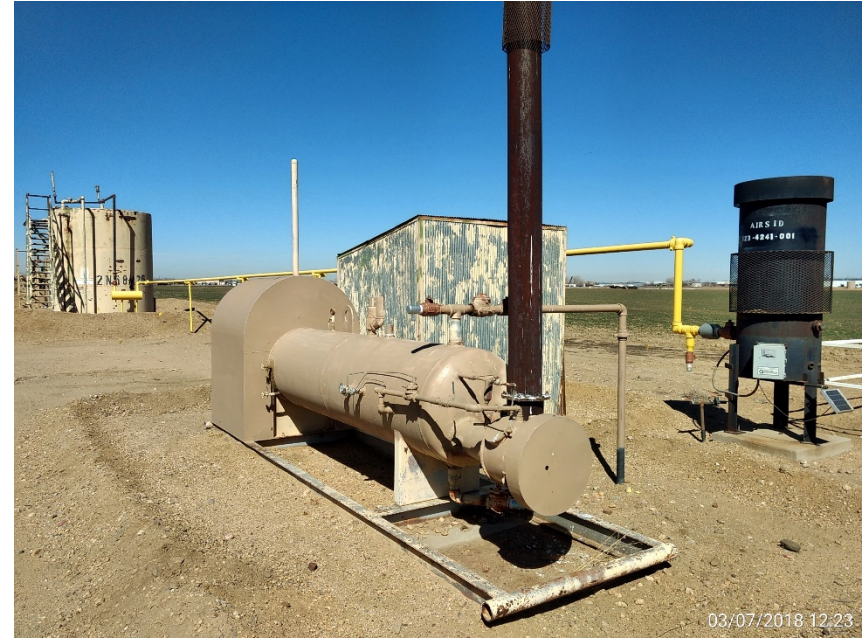
Separator, ECD, & Manifold housing
