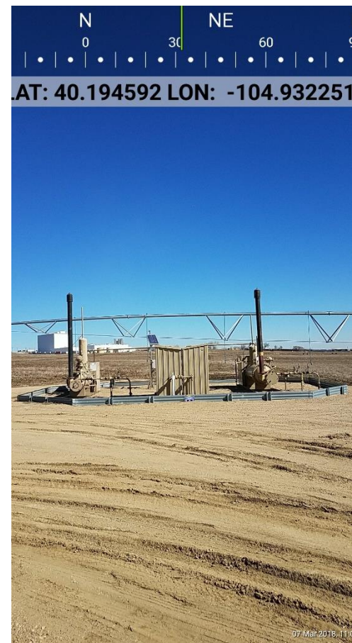
Photo 3 Separators and Gas Meter Runs
