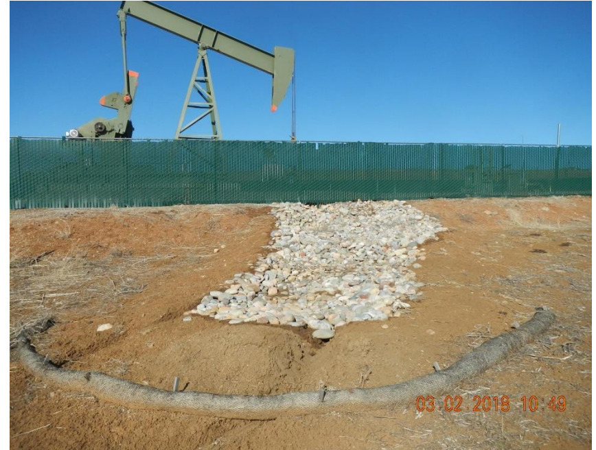
Rip rap and wattles on eastern edge of location.
