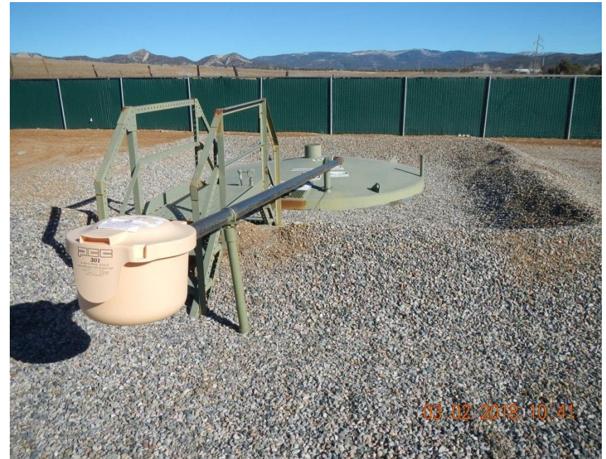
Drip pot on load out line.
