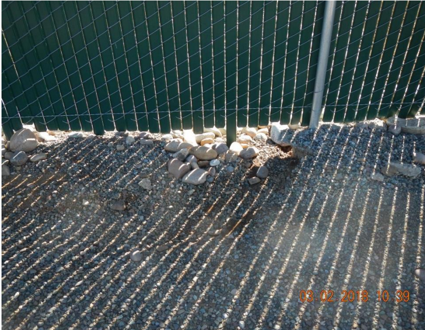
Erosion along eastern edge of location.
