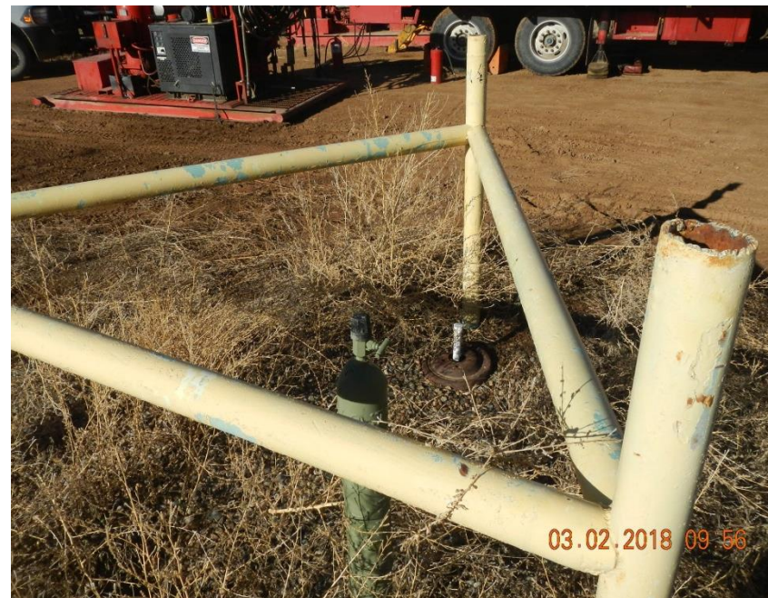
PA marker for Hill #1-8 with PVC soil vapor tube.
